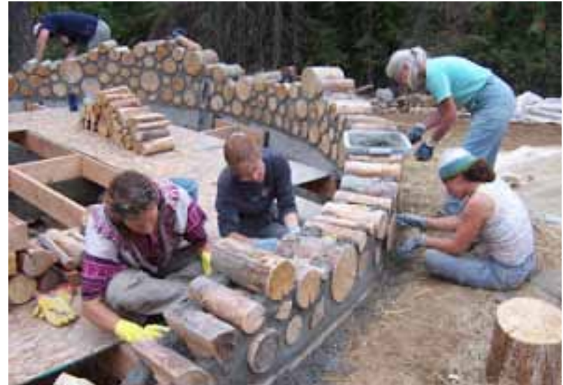
Fig. 10.14 - Curved stackwall construction.
