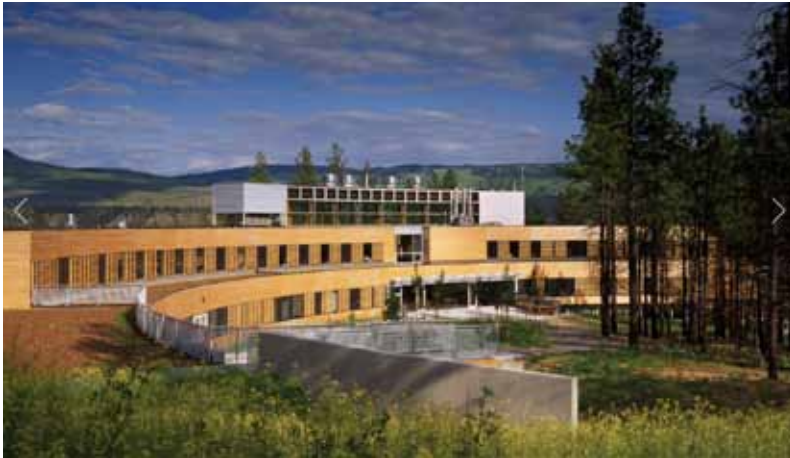
Fig. 4.22 - The semi-circular cedar-clad shape of the Nicola Valley Institute of Technology emerges from forested south-facing slope blending with the site.
