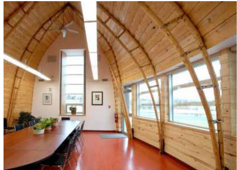
Fig. 10.15 - Bent pole trusses + wood decking inspired by Pictou Landing Health Centre (Richard Kroeker Design)
