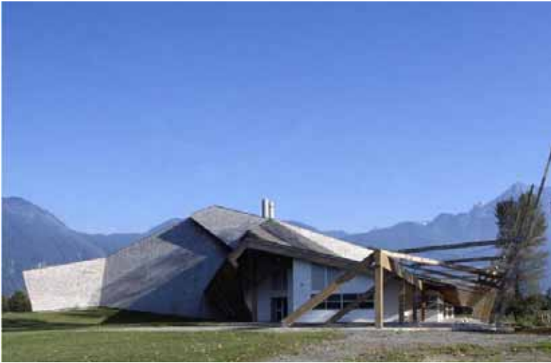
Fig. 4.24 - Building form responds to climatic conditions, closed to the north + west mimicing the mountainous backdrop and open to the south + east.
