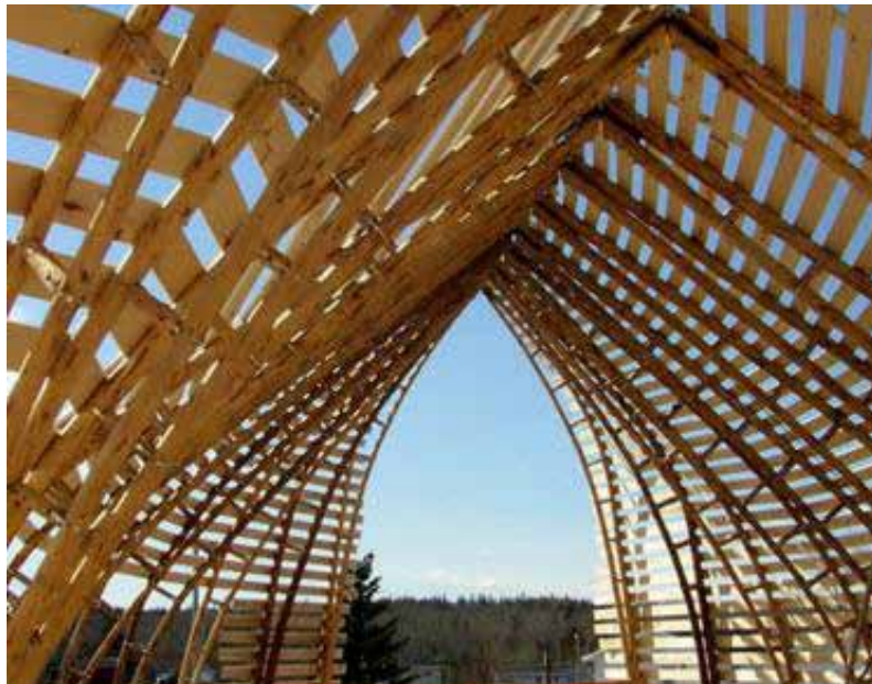
Fig. 4.30 - Bent pole trusses form a light-weight sinuous vaulted space.
