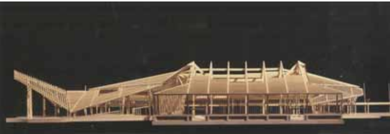
Fig. 4.25 - Seabird Island School 1:50 wood framing model.
