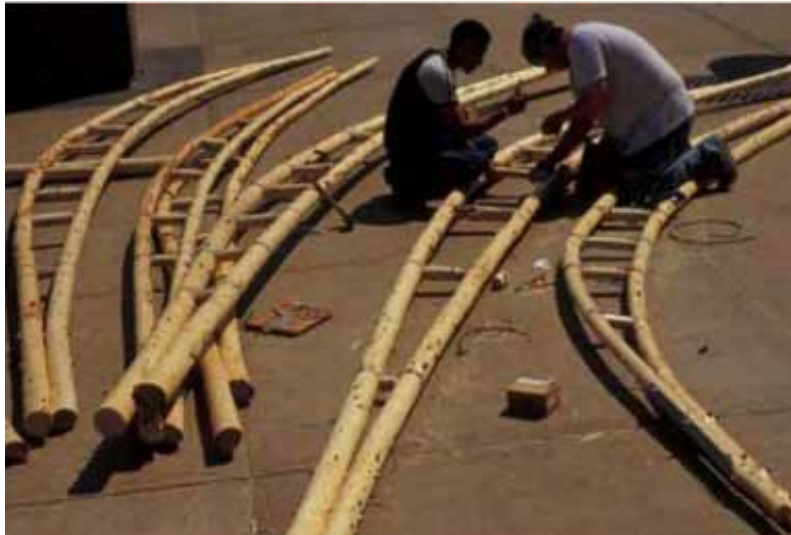
Fig. 4.29 - Bent pole trusses assembled by the Pictou Landing First Nation.
