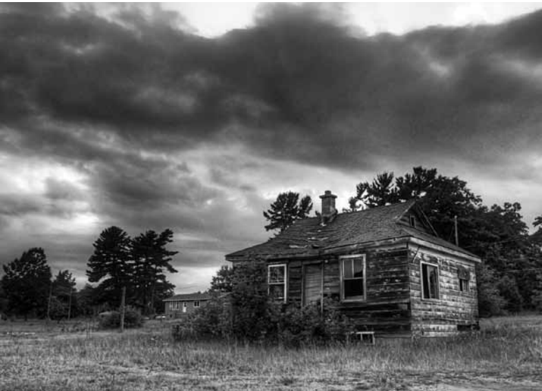
Fig. 7.10 - Remains of a settlement house as of 2011.
