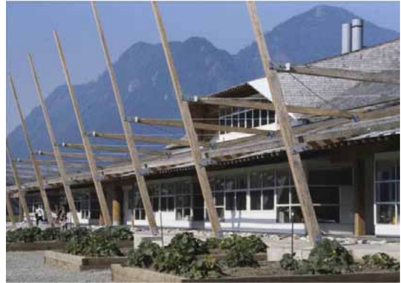
Fig. 4.27 - The use of a variety of struts, beams and trellises echoes the totemic elements associated with early styles of West Coast architecture. Also shown are the south facing classrooms opening out to the teaching gardens.
