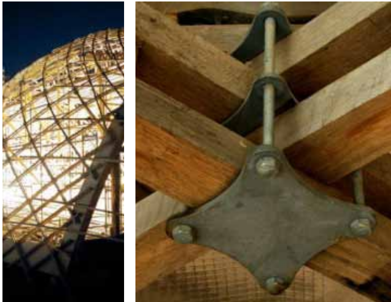
Fig. 10.17 - Gridshell construction domical form and connection as inspired by the Weald and Downland Open Air Museum
