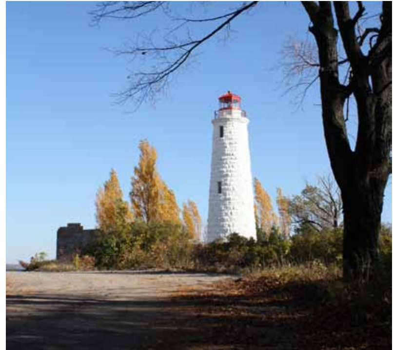
Fig. 9.24 - Christian Island lighthouse and light keeper house ruins in 2011.
