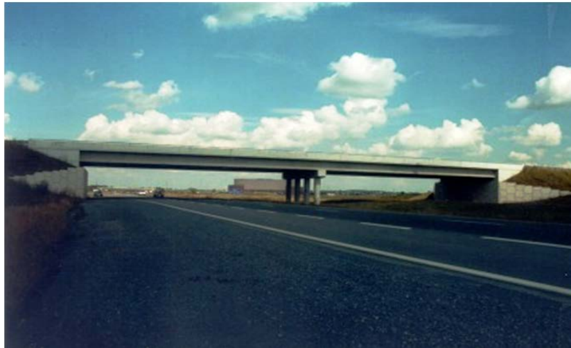
Figure 3.3: Elevation View of Palladium Drive IAB (Husain & Bagnariol, 2000)
