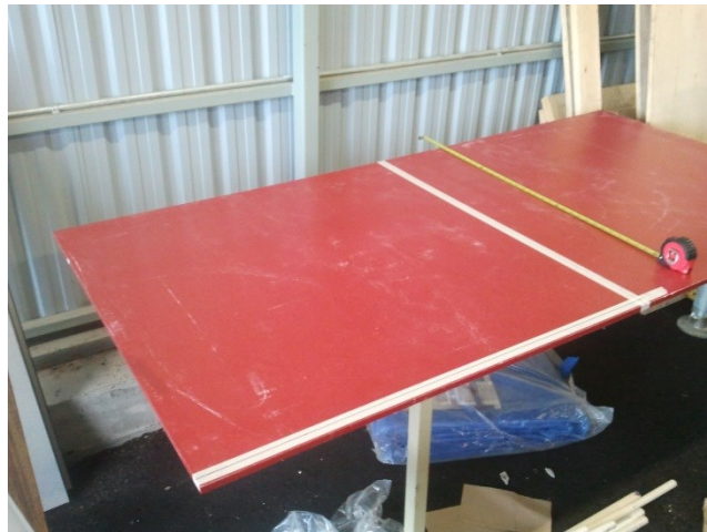
Figure 3-9: Base layer fiberglass cutting
