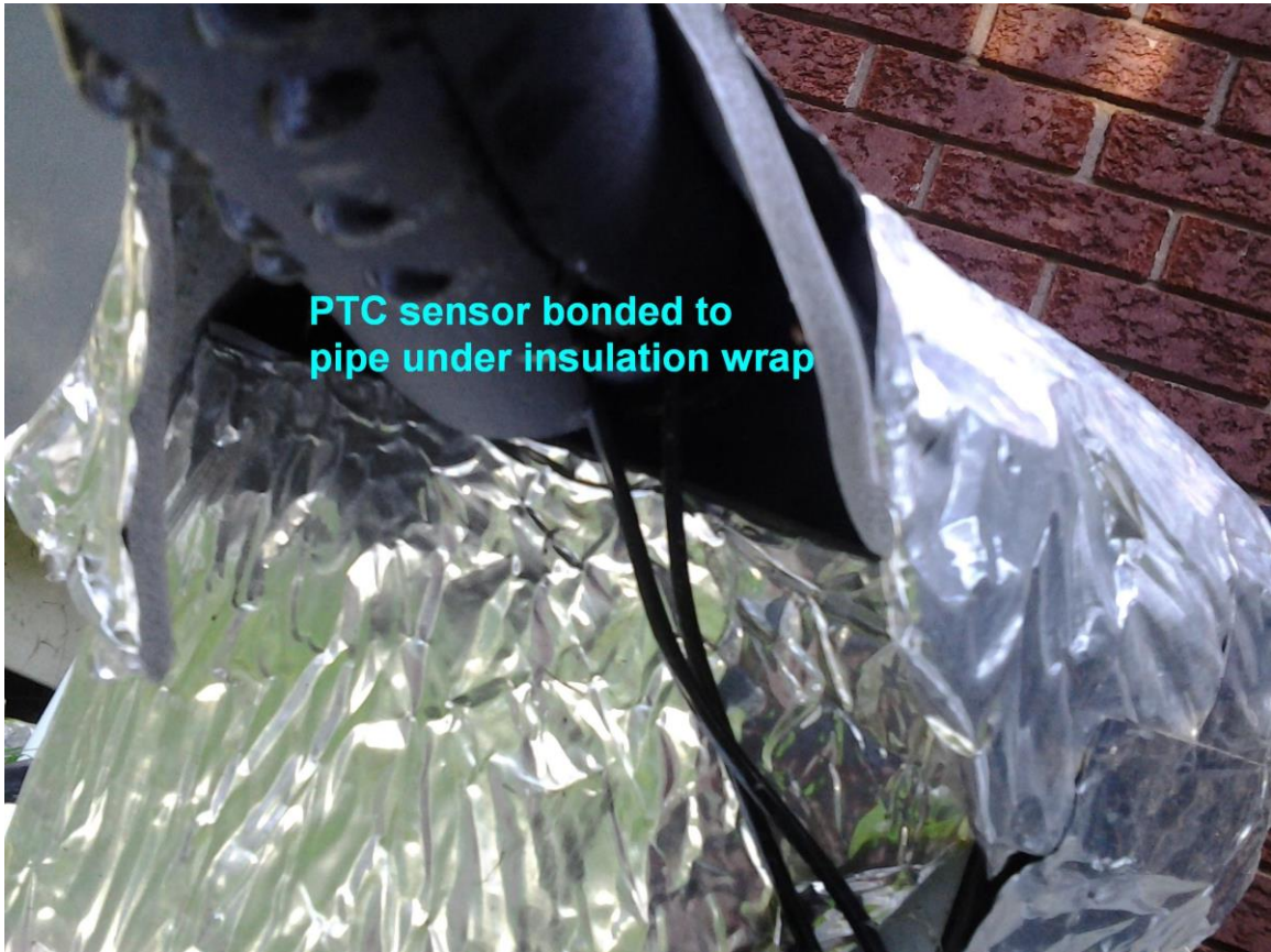
Figure 18 – Photo of Compressor Thermal Protection Placement
