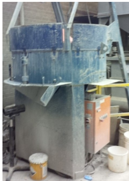
Figure 3.9: Concrete mixer used for concrete production
