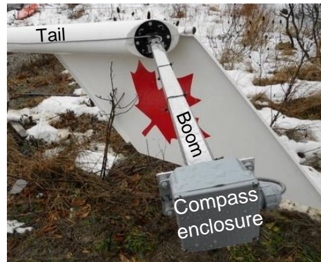
Figure 3.13: Mounting of digital compass yaw sensor on an aluminum boom to reduce magnetic interference with the compass. (Wind turbine in its lowered position.)
