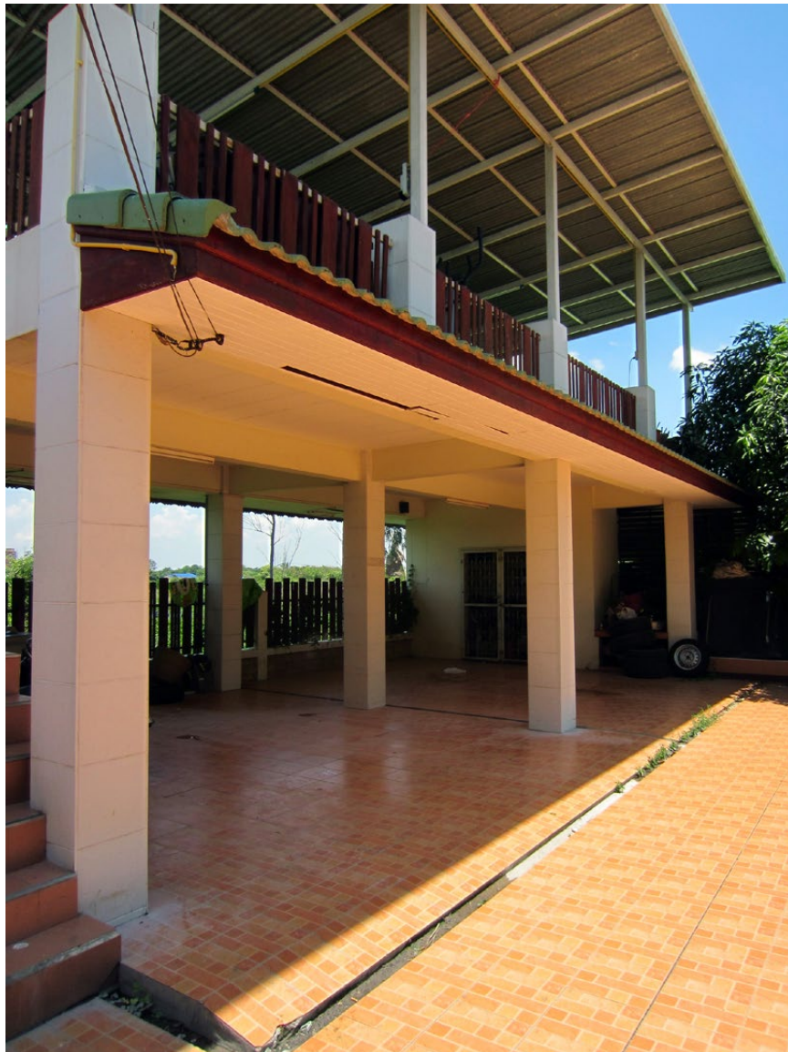
the back of Note's home which looks out onto the marsh
