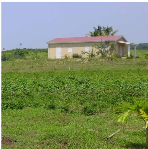
View of training facility at Agro-Tourism Farm
