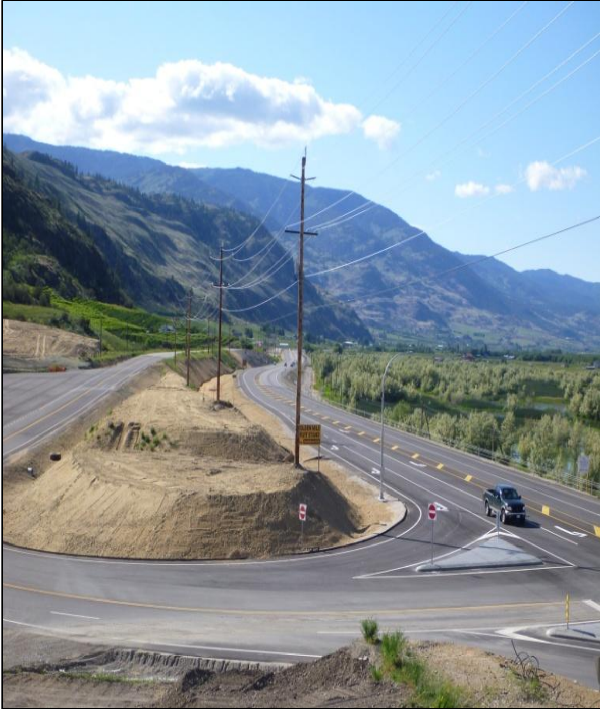
Figure 2. Osoyoos Passing Lanes (OPL transect) prior to fencing installation and interchange to frontage road (completed, 2011); Northwest facing photo. Straight-line distance from upland (westward) frontage road ditch slope across to (eastward) lowland floodplain is approx. 108 m. Photo credit J. Crosby 2012.
