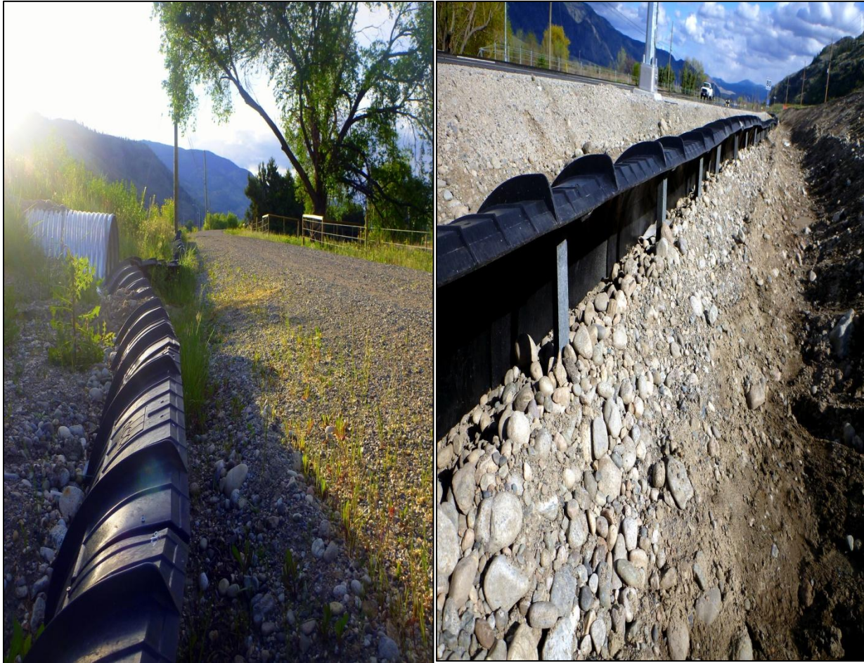
Figure 5. Permanent ACO polymer plastic amphibian fencing along the Hwy 97 Osoyoos passing lanes area. Left photo: Fence line connecting to the ‘Ponds’ culvert, adjacent to a bike path. Right photo: fencing when first installed west of Hwy 97 across from the No. 22 road.
