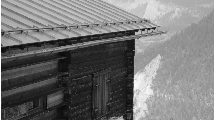
figure E.03 Zumthor's House Truog Gugalun in Versam, Switzerland, 1994: juxtaposition of old and new construction
