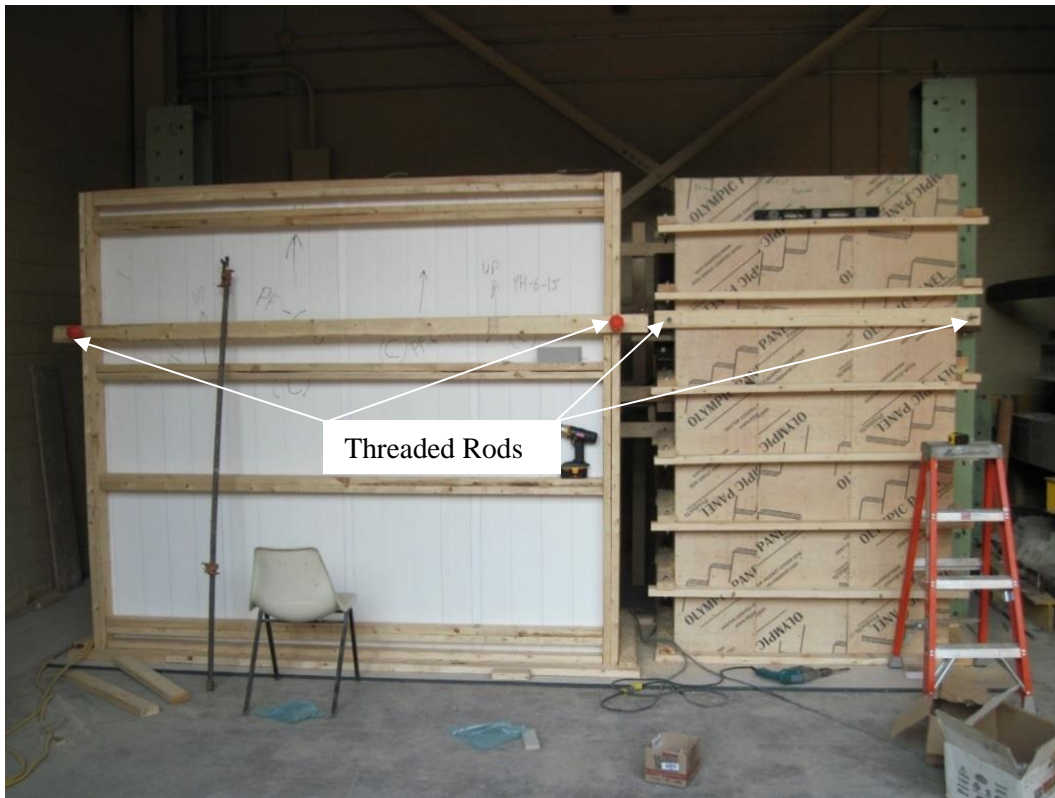
Figure 3.6: Specimens in place before casting
