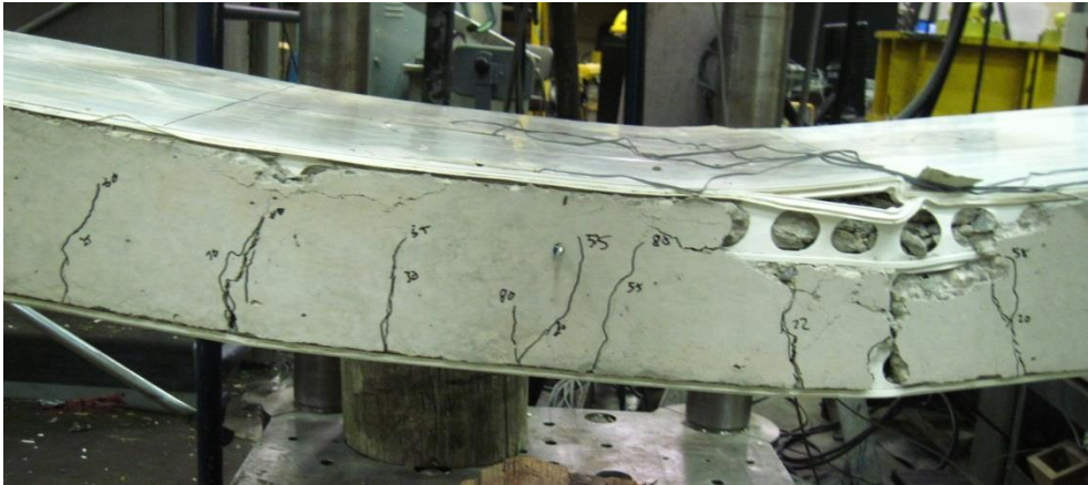
Figure 5.11: Failure at right loading point for wall PH-6-15.
