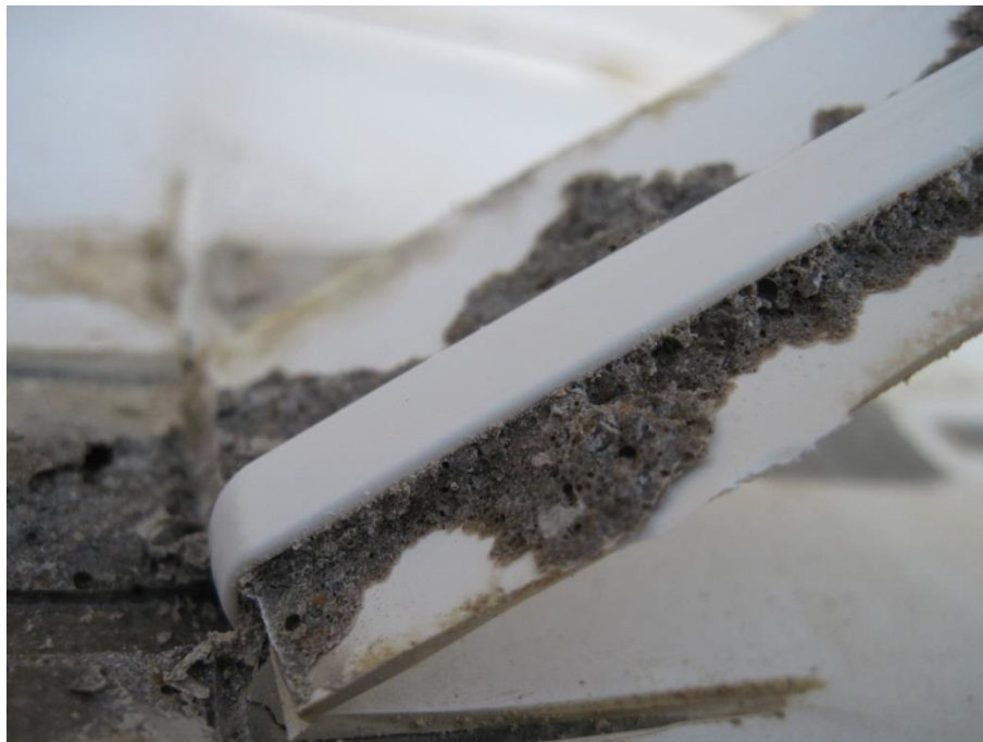
Figure 4.32: Concrete paste attached to PVC ‘nubs’.
