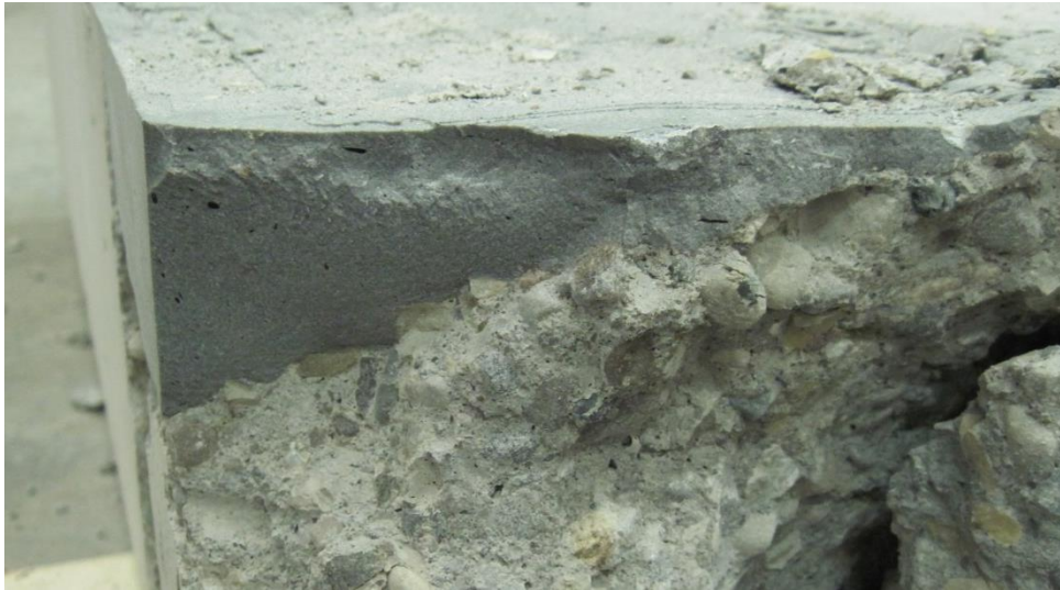
Figure 3.10: Evidence of bond achieved between concrete and patch material.
