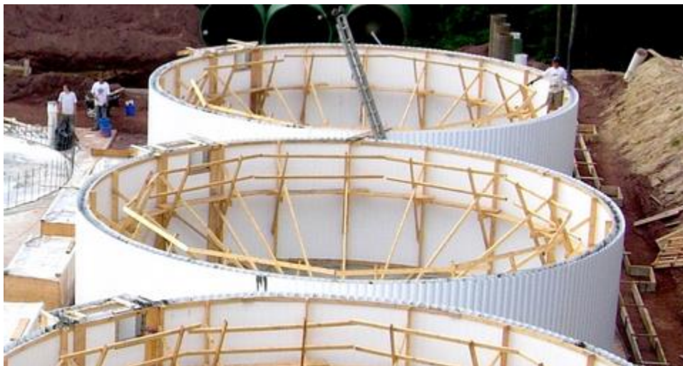
Figure 1.1 Example of tank construction using SIP formwork
