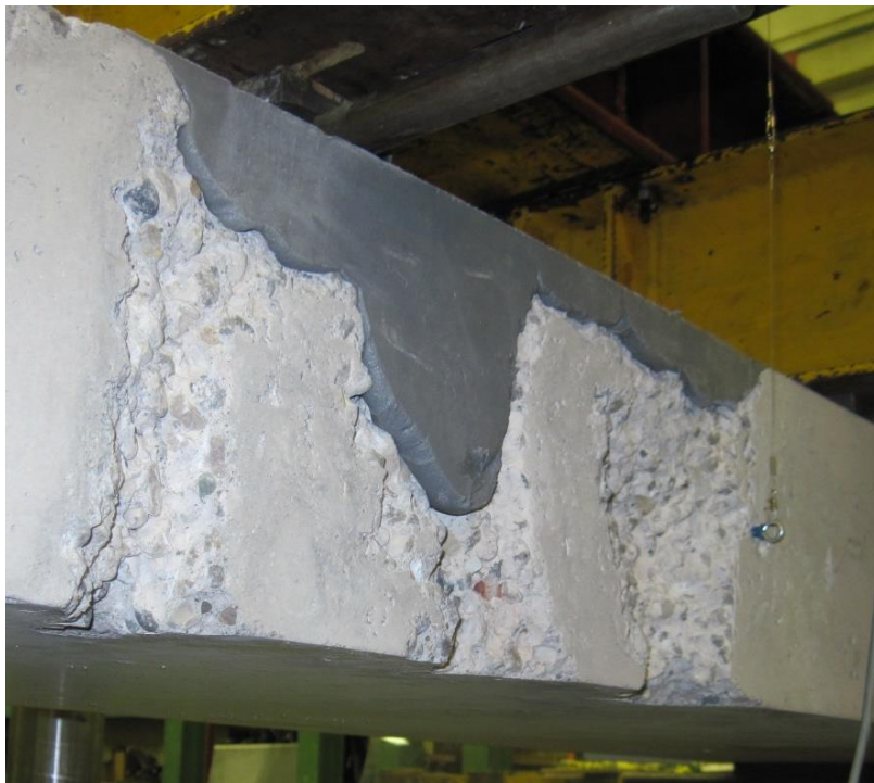
Figure 3.9: Example of patch material applied to concrete wall with segregation.
