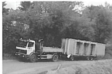
Transport of wall elements
