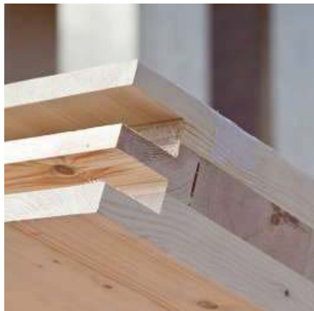
Fig. 3.6 (Top) Half-lapped panel-to-panel connection. Photo by CrossLam Timber Solutions LLC.
