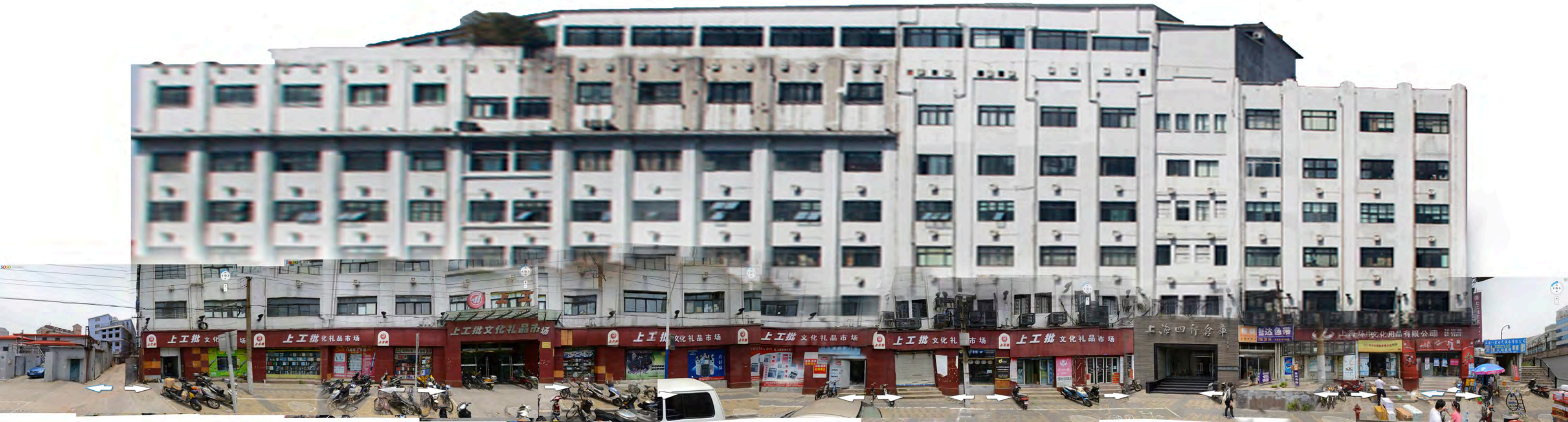
Fig 4.7 Collage of the south elevation made of about forty photos.
