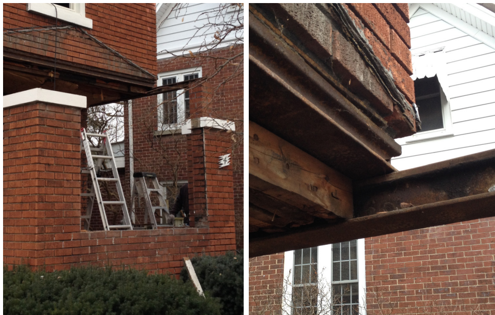
Fig. A.2.3.d. Original Connection
