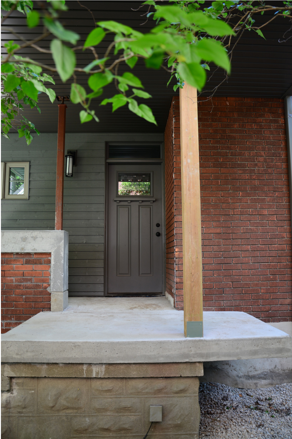
Fig. 6.1.l. Front Door Just the railing yet to be installed.
