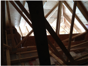
Fig. A.2.4.e. Insulation Baffle
