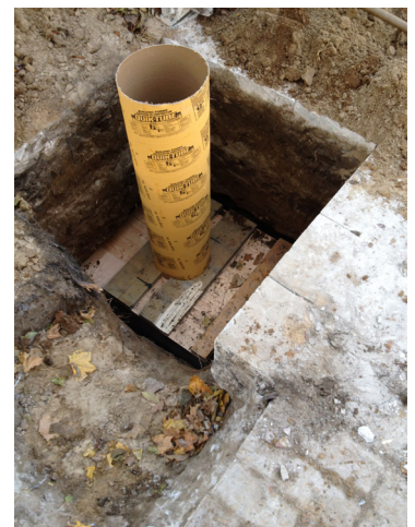
Fig. A.2.2.e. The Hole with Formwork
