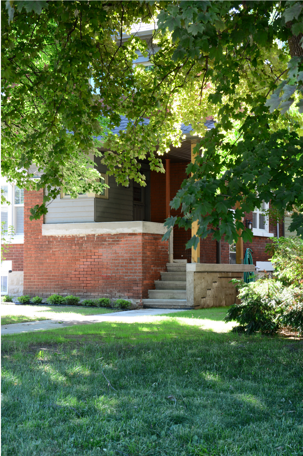
Fig. 6.1.j. Queen Street Approach
