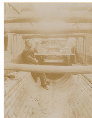
Figure 2.2 [below] Building of the first Garrison Creek Sewer. 1890s.
