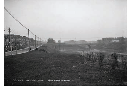
Figure 1.8 Bickford Park, looking south, with Harbord bridge in the distance.
