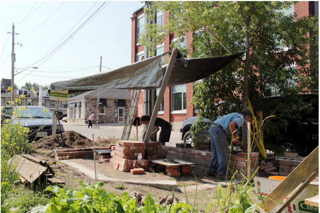
[xxviii] School greenhouse building in progress.
