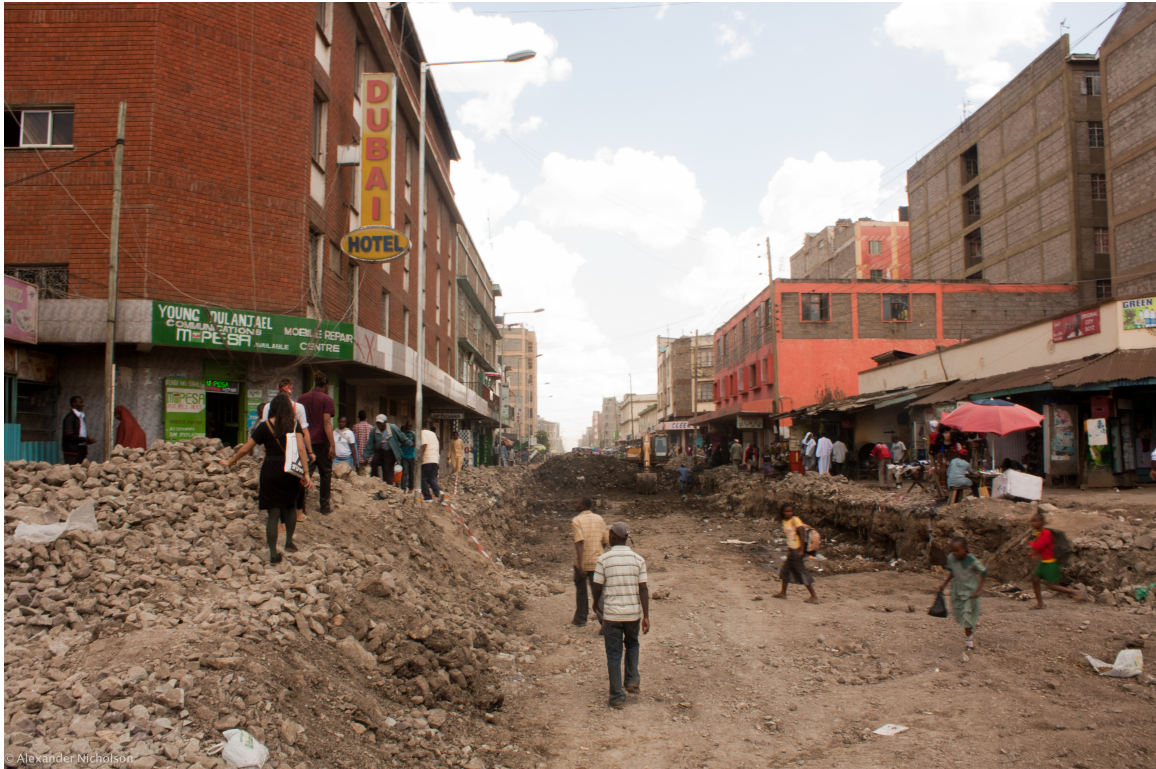
Figure 4: Unfinished Road near First Avenue in Eastleigh
