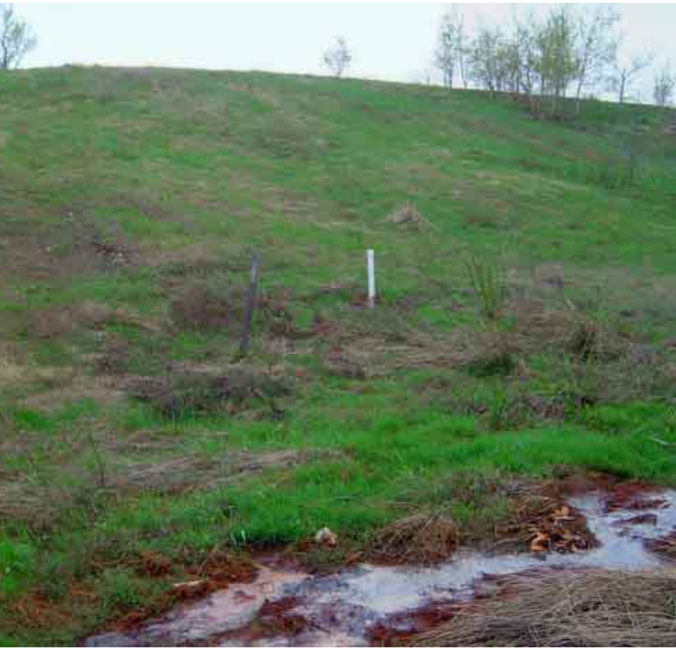
fig. 1.11 leachate pooling around perimeter of the petitcodiac riverside landfill
