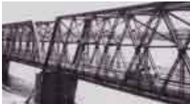
fig. 2.9 gunningsville bridge, built for horse and carriage, 1907
