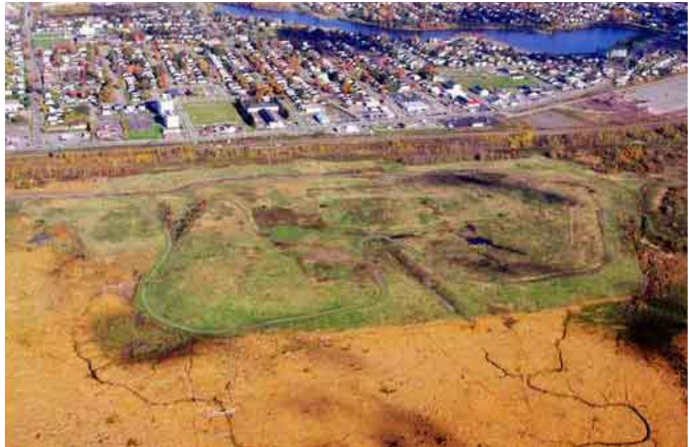
fig. 2.53 landfill mounds built up on the marshes of the petiscodiac river. distressed vegetation and leachate seepage around perimeter visible
