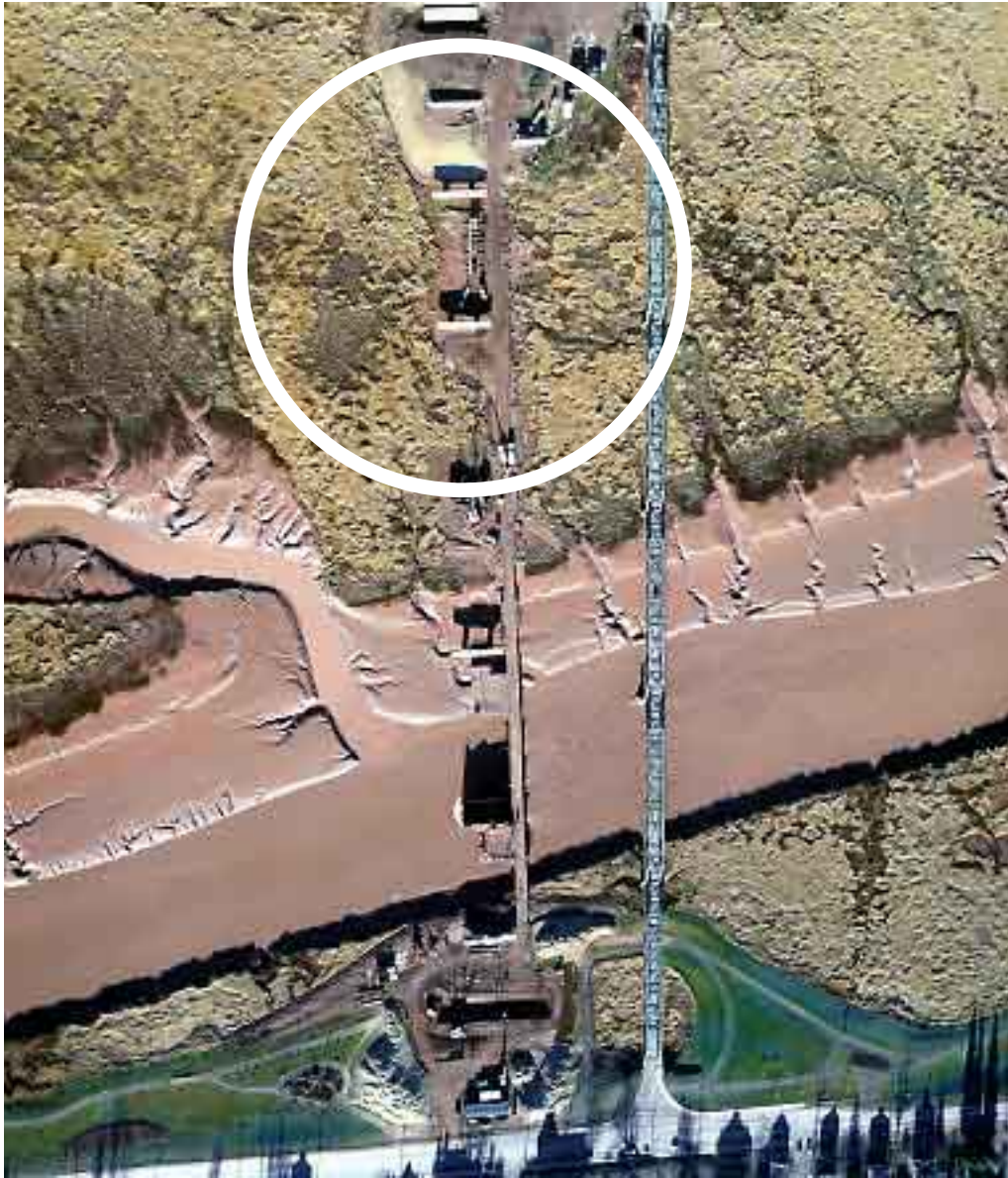
fig. 2.20 the last remaining 40 acres of the original Jonathan Creek disappearing with the ongoing construction of the new Petitcodiac River bridge approaches, 2005
