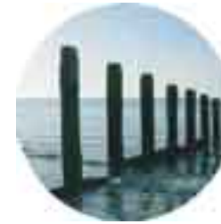
fig 3.77 groyne, low tide
