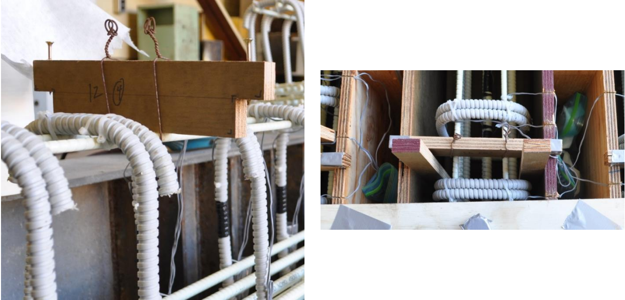
Figure 3.6: Collection of Rebar Blocking Photos
