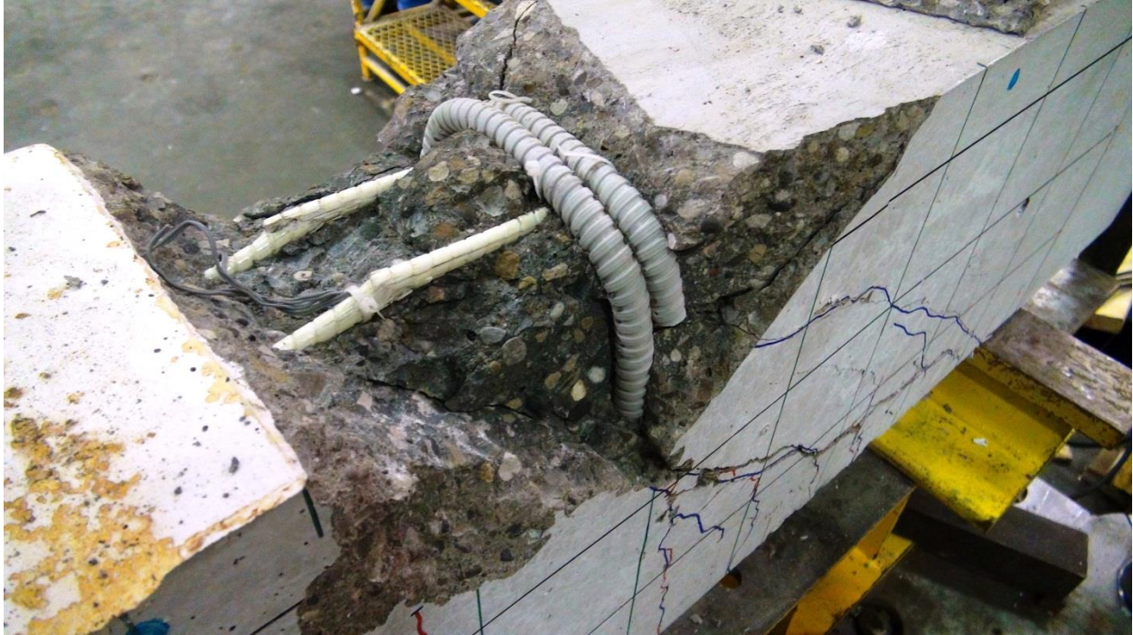
Figure E.66: BM12-220 Photo of Exposed Stirrup 7 after Testing
