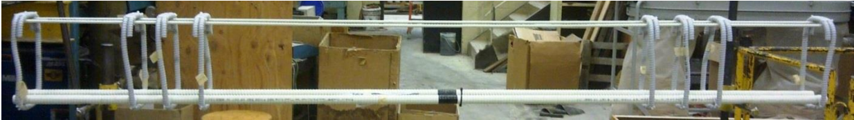
Figure E.44: BM25-INF Rebar Cage Elevation Photo
