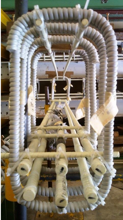
Figure E.31: BM16-INF Rebar Cage Cross-Section Photo
