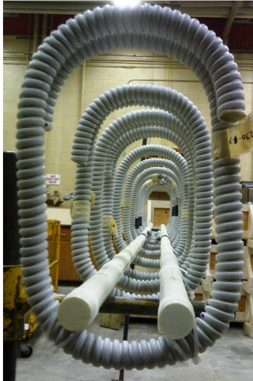
Figure E.246: BM25-s230 Rebar Cage Cross-Section Photo Top framing bar not pictured.
