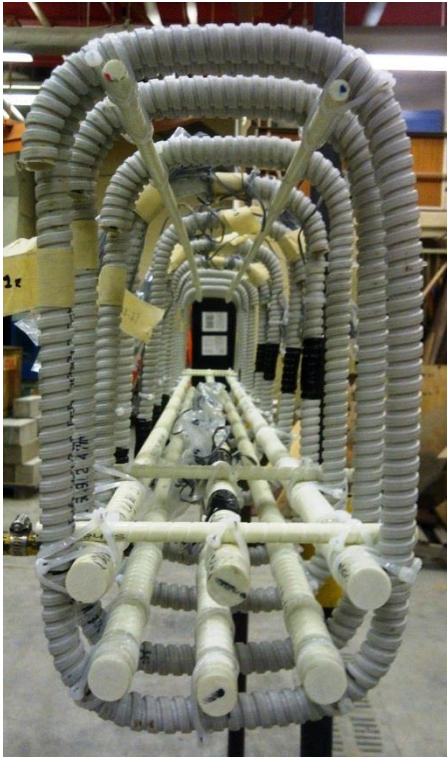
Figure E.89: BM16-220 Rebar Cage Cross-Section Photo
