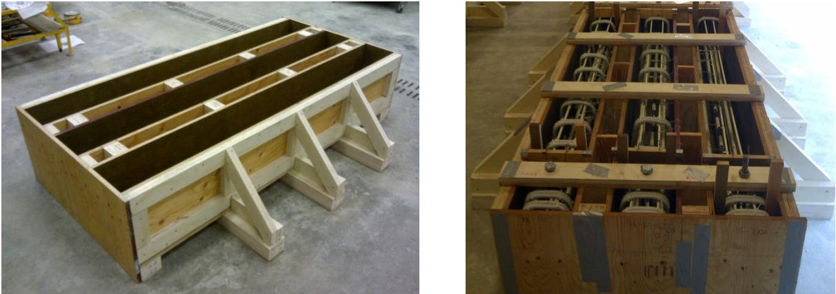
Figure 3.5: Collection of Formwork Module Photos for the Group 16 Beams
