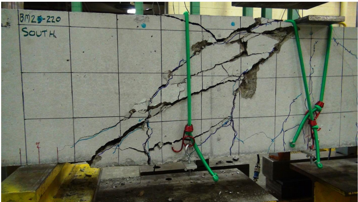
Figure E.113: BM25-220 Close-up Photo of Failure
