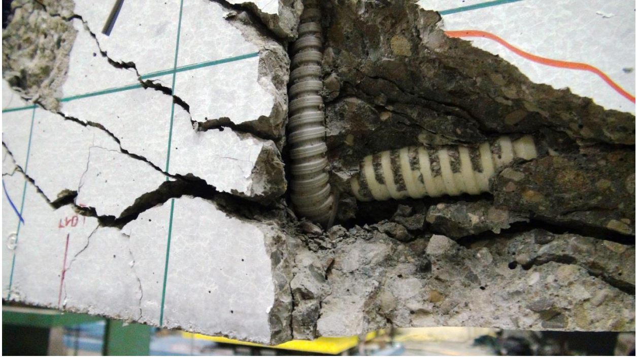
Figure E.114: BM25-220 Photo of Exposed Stirrup after Loading 1
