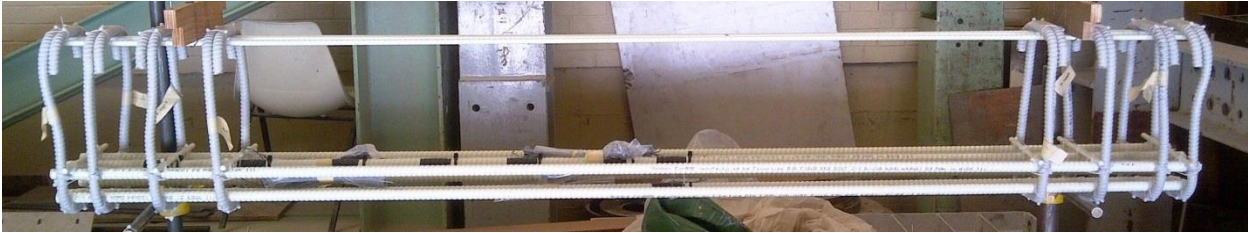
Figure E.30: BM16-INF Rebar Cage Elevation Photo
