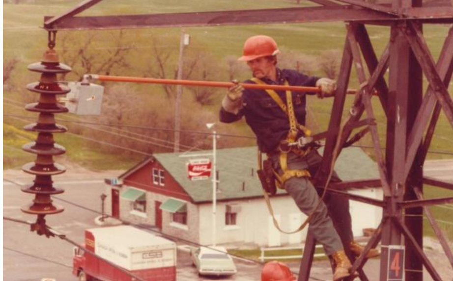
Figure 1.10: Hi-Pot Field Test.
