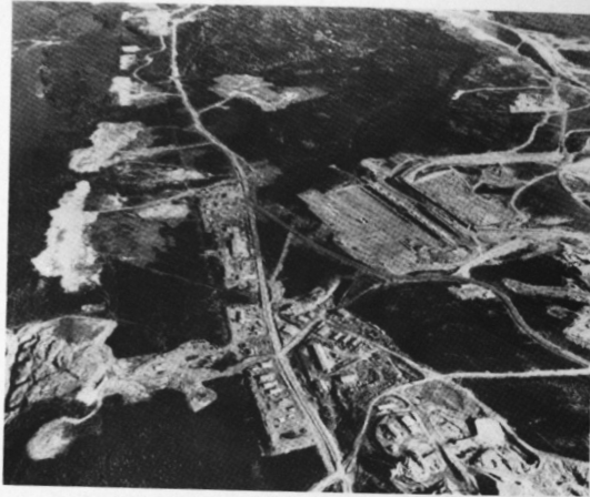
James Bay. First of three power plants under construction. First phase of La Grande Complex to be completed by 1995. Courtesy of UPI/Bettmann.
