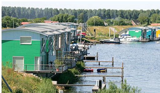
Figure 4.66 Floating houses of Maasbommel
