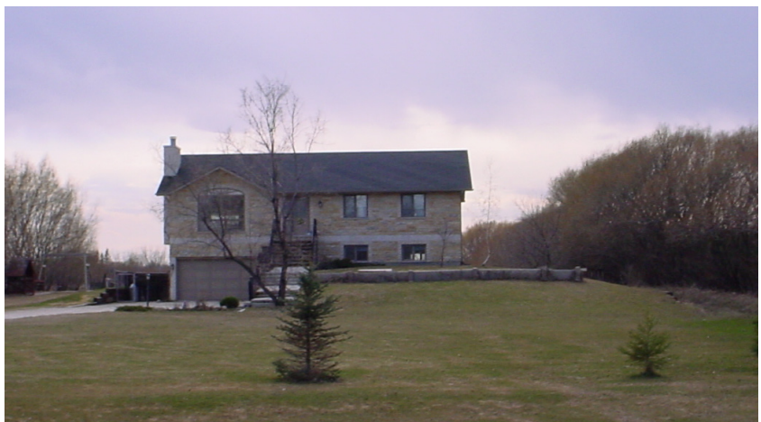
Figure 3.12 House on hill, with garage partially displacing fill
