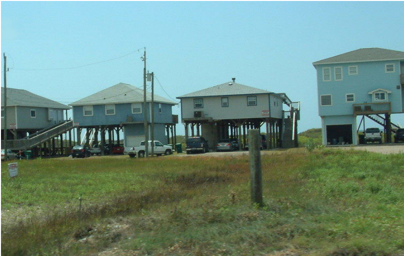
Figure 4.93 Houses on stilts on the outskirts of Houston, Texas, built for hurricane force floods
