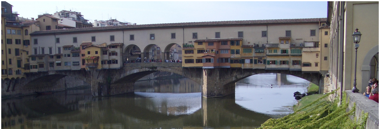
Figure 4.25 Ponte Vecchio in Florence, an early megastructure
