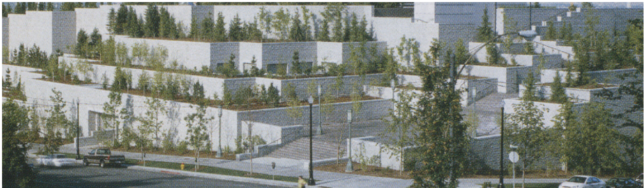
Figure 4.46 Landscaping effect, planned by stepping the apartments on the south, west and east sides.
