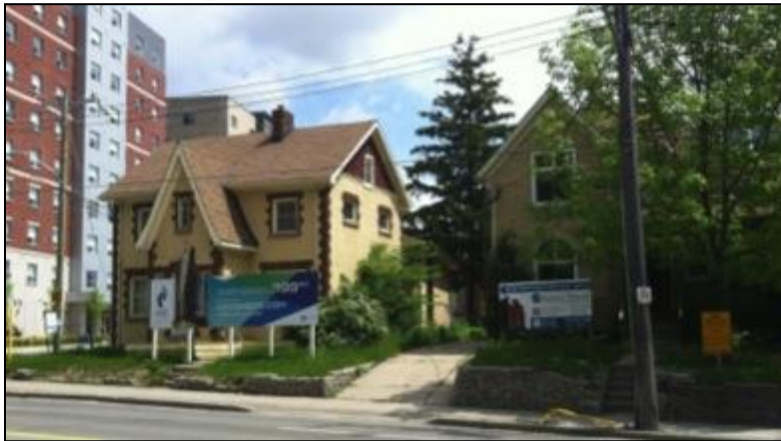
Figure 8 - Example of a residential land assembly along the Uptown Corridor
