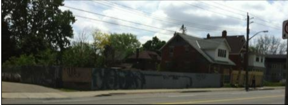
Figure 20 - Example of poor interim land assembly conditions in Uptown Waterloo
