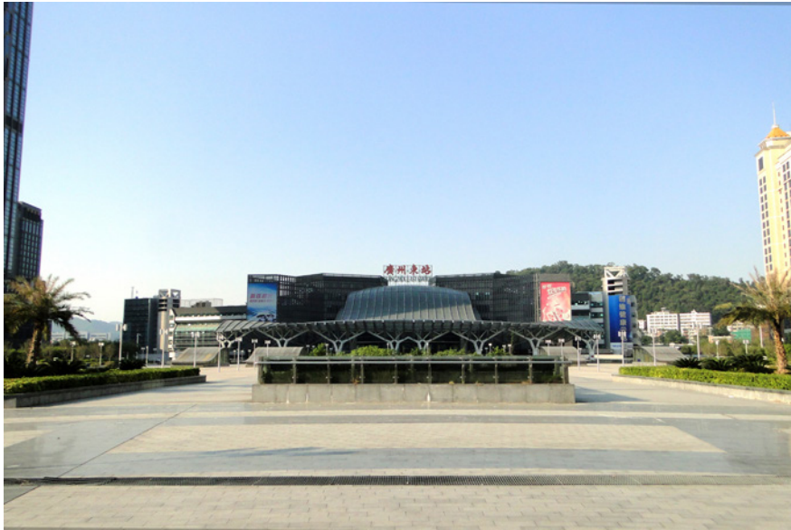
Fig2.24 Guangzhou East Railway Station
