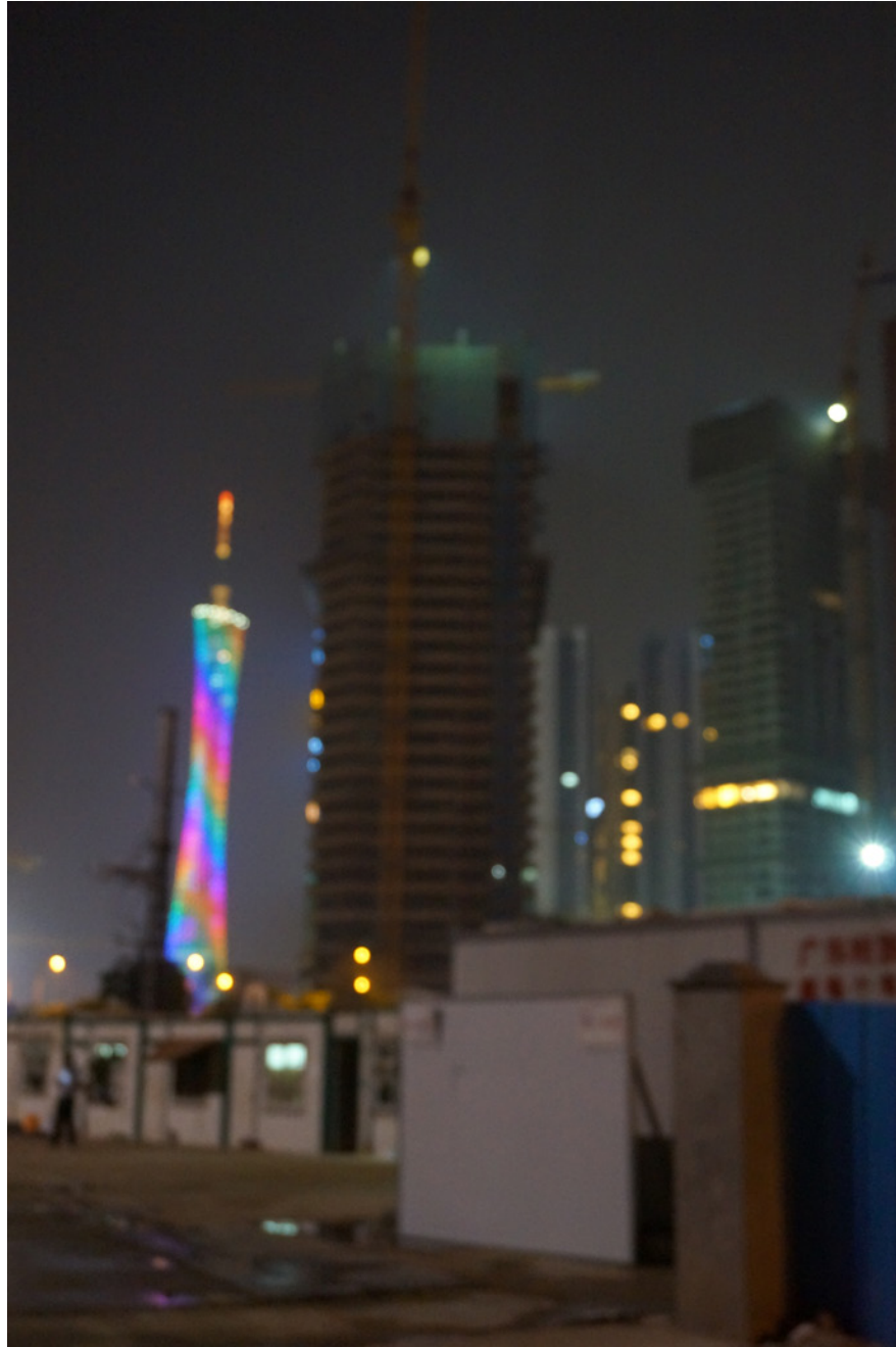
Fig2.39 Construction Site of Liede Village
