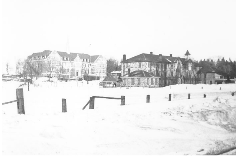
5.11 The new Shingwauk IRS being constructed behind the old, 1934-35
