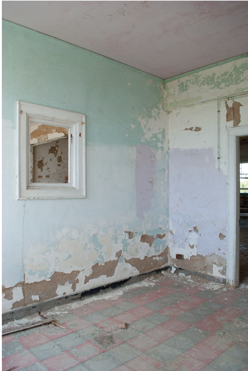
3.16 Monitor overlooking second-floor boys' dormitory, Birtle, 2013
