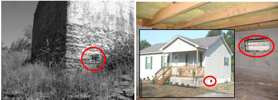
Figure 2-3: Vents for Crawl Spaces
