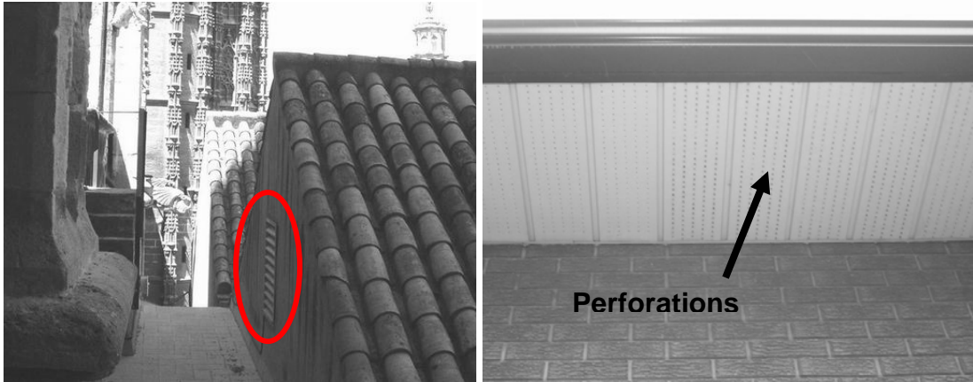
Figure 2-5: Attic Vents
