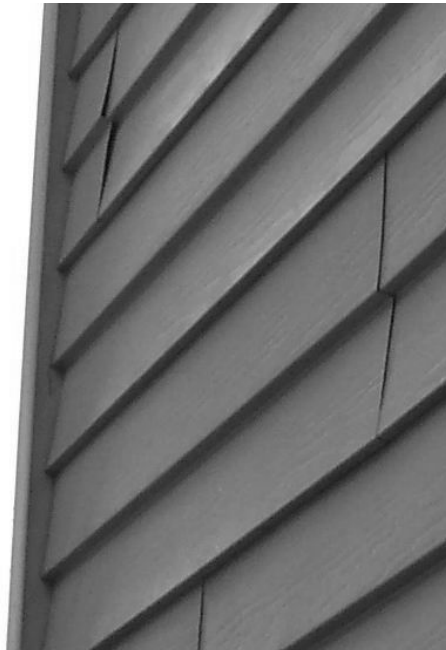
Figure 3-32: Typical Installation of Vinyl Siding (Waterloo, Canada)
