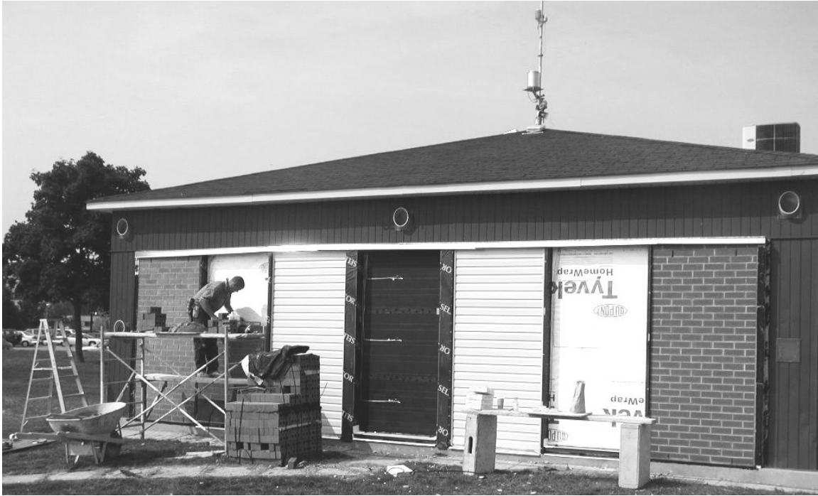
Figure 8-1: Mason Installing a Brick Veneer after Instrumented Panels are installed
