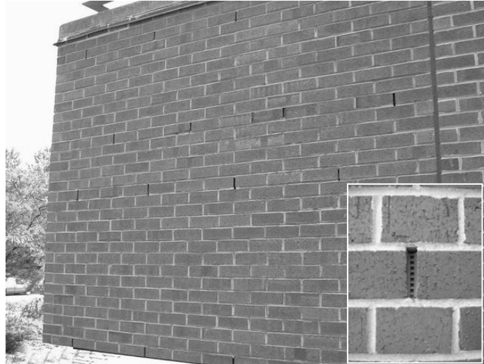
Figure 3-22: Repaired Ventilated Brick Veneer (Hagey Hall – Waterloo)
