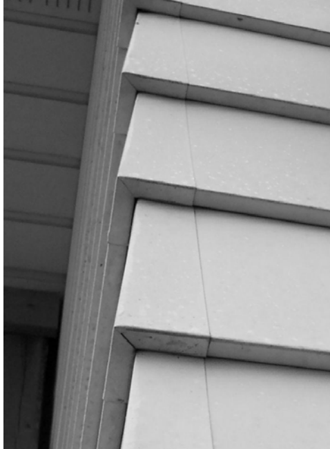
Figure 3-31: Typical Installation of Aluminum Siding (Waterloo, Canada)
