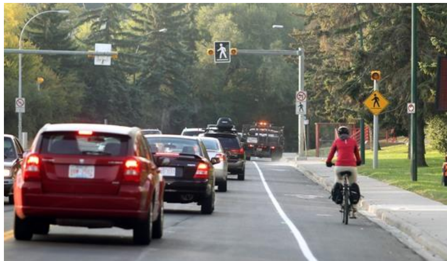
Figure 4: Road with Dedicated On-Road Bike Lane (Source: www.blogs.calgaryherald.com )
