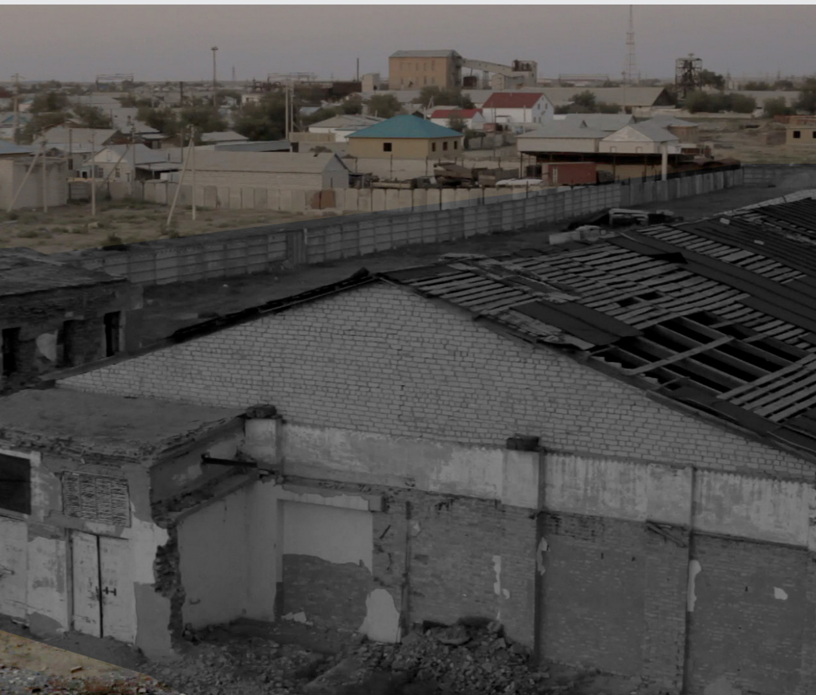
FIG. 92 Industrial ruins (foreground) and new homes (background) in Aral'sk.
