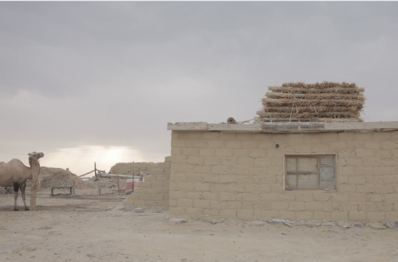
FIG. 73 Vernacular building materials, sourced locally: mud bricks, straw/reed mats, wool from livestock.
