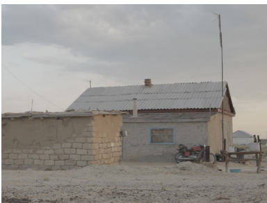
FIG. 84 Mud brick building finished with an outer coat of paqsa .
