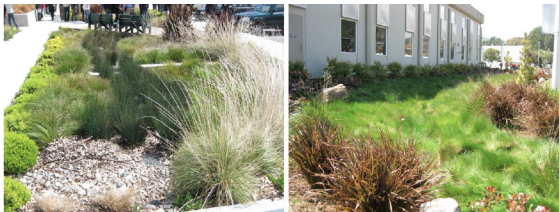
Left: Fig. 12. Rain garden, Police Department, City of Brisbane, California, USA (© J. Hoyer). Right: Fig. 13. Swale, Police Department, City of Brisbane, California, USA (© J. Hoyer).
