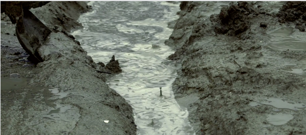
FIG. 16 During spring thaw (in late March), a period of heavy rains and flash-flooding, residents dig trenches to prevent their homes from flooding.
