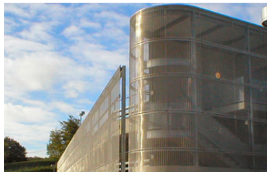
FIG. 60 Mesh cladding on Cork County City Hall, Eire
