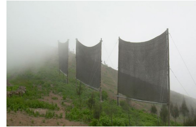
FIG. 42 Fog collectors in the hills near Lima, Peru harvest water from prevailing winds for a region that experiences less than 1.5cm of rainfall per year.
