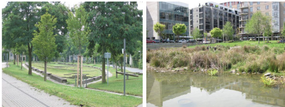
Left: Fig. 14. Detention pond (dry), Gelsenkirchen, Germany (© J. Eckart). Right: Fig. 15. Detention pond (wet) in Tanner Springs Park, Portland, Oregon, USA (© J. Hoyer).
