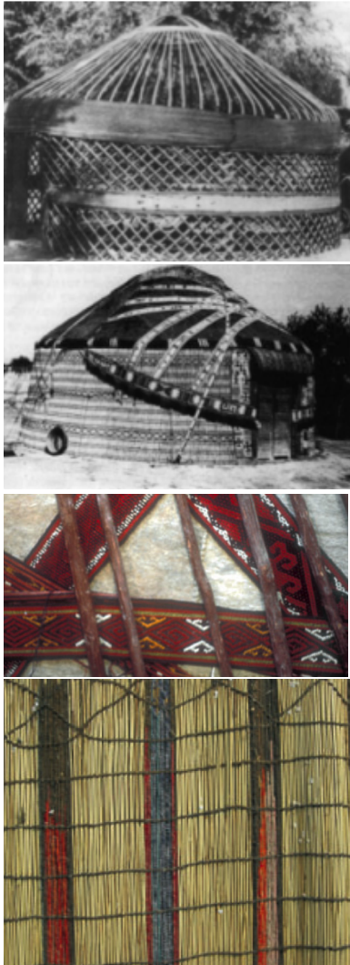
FIG. 76 Layers of the Kiiz Ui : a wood scaffold, lined with felt and reed mats
