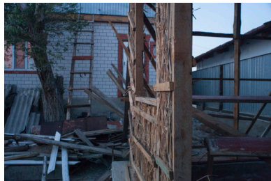
FIG. 83 The construction of a summer house, filled with straw/reed walls
