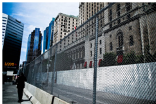
A.9 BAY & FRONT | FLICKR The construction of the fence is complete.
