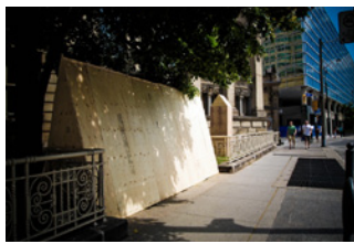
A.8 DOWNTOWN | FLICKR Monuments adorning Front St. are covered in plywood.
