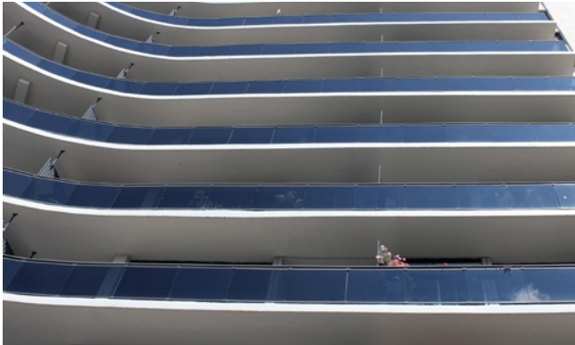
Figure 1-11 Typical Balconies: 1970s (Renovated)
