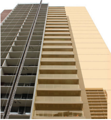
Figure 2-4 Extension to 66 Isabella Street, Toronto: Currently Under Construction
