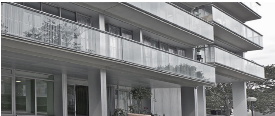
Figure 2–25 left The Addition of the Extended Balcony and the transformation of the dated tower: Lacaton and Vassal, Paris.
