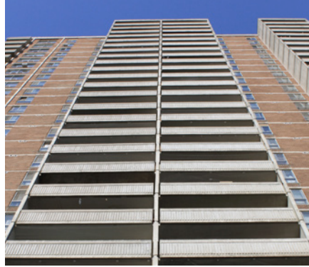
Figure 5-16 565 Sherbourne Street: East View
