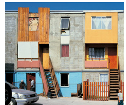
Figure 1–3 top Intended Informality: Quinta Monroy Housing, Elemental, Chile (2004). The provided framework for adaptation.
