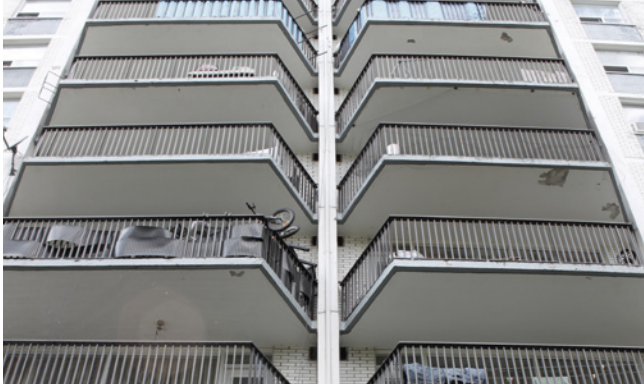
Figure 1-7 Typical Balconies: 1960s
