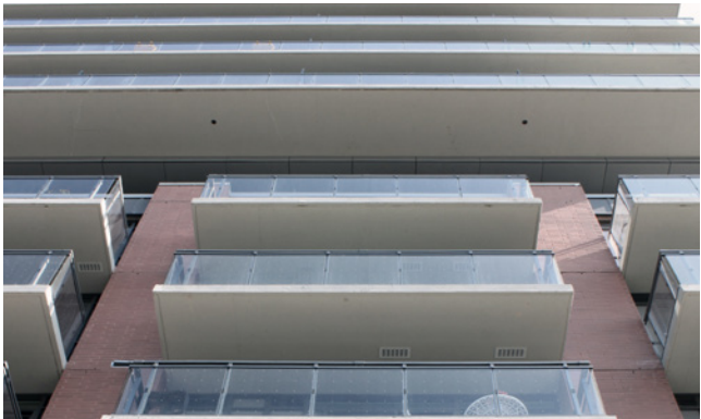
Figure 1-13 Typical Balconies: 2010s
