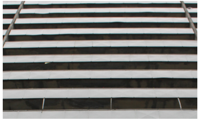
Figure 1-10 Typical Balconies: 1970s
