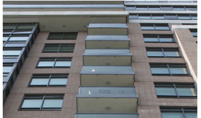
Figure 1-14 Typical Balconies: 2010s
