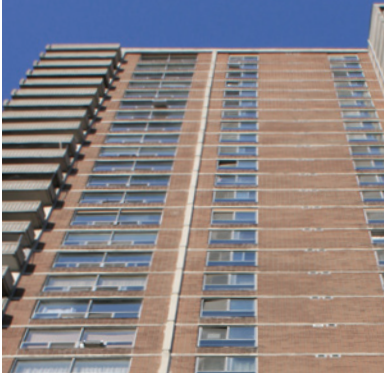
Figure 5-15 565 Sherbourne Street: East View
