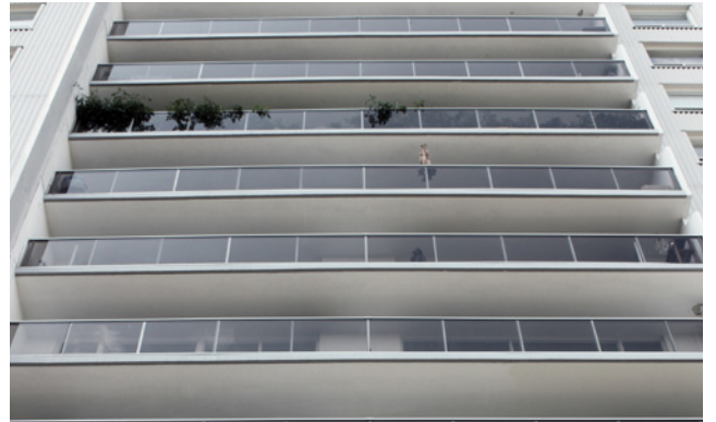
Figure 1-12 Typical Balconies: 1970s (Renovated)
