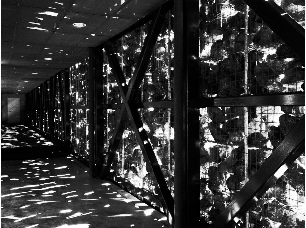
Fig 2.33 Dominus Winery gabion wall
