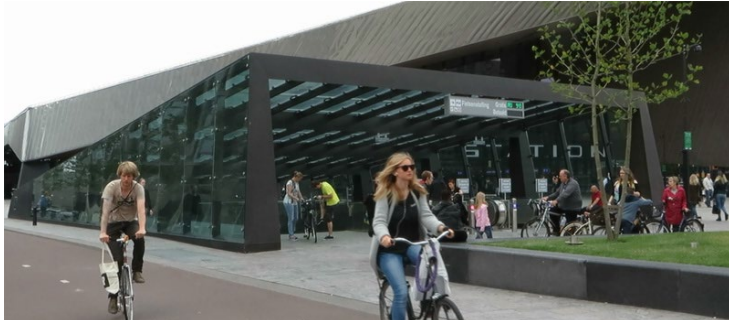
Figure 4-19 Rotterdam Central Station bicycle entrance
