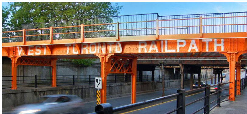
Figure 3-30 Bridge over Bloor St. West
