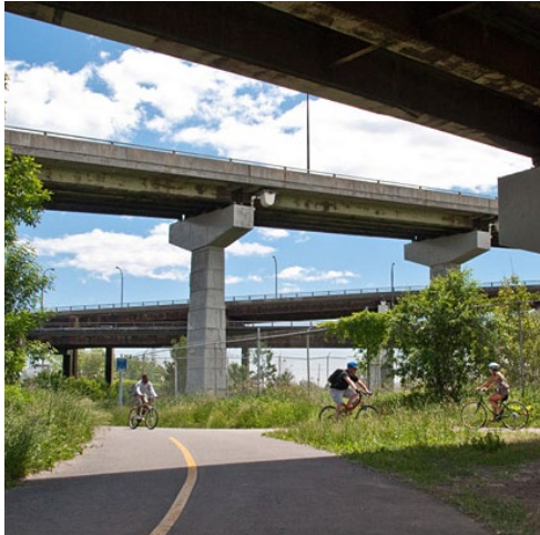
Figure 3-25 Below the Gardiner Expressway ramps
