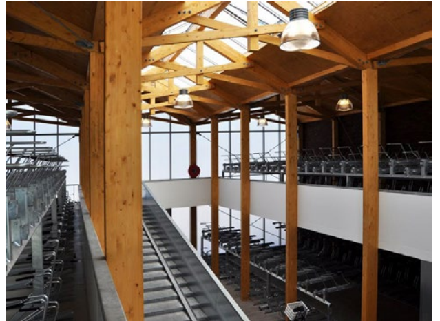
Figure 4-8 Bicycle Warehouse interior
