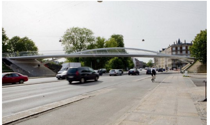
Figure 4-40 Agade Bridge cyclist crossing
