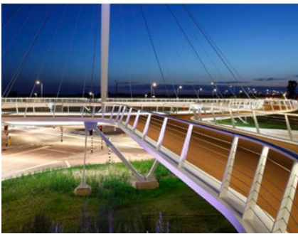
Figure 4-34 Hovenring Bridge separation
