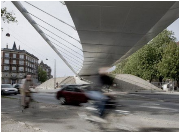
Figure 4-39 Agade Bridge underside
