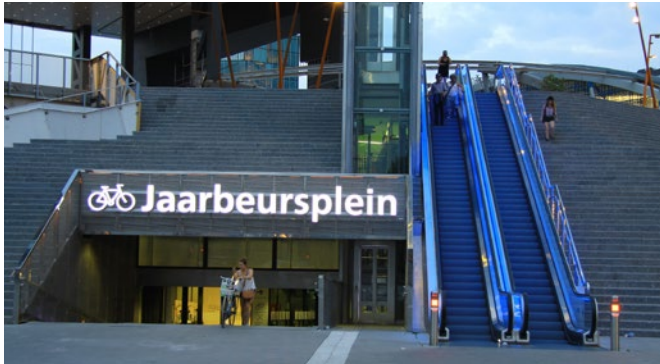
Figure 4-25 Utrecht Central Station bicycle entrance
