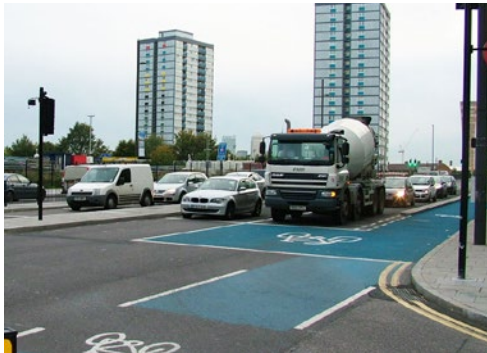
Figure 3-14 Bike box intersection
