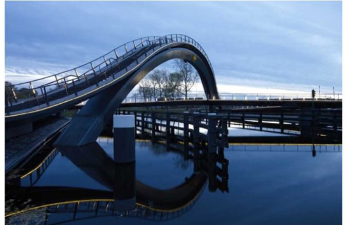
Figure 4-38 Melkweg bridge pedestrian and cyclist canal crossing
