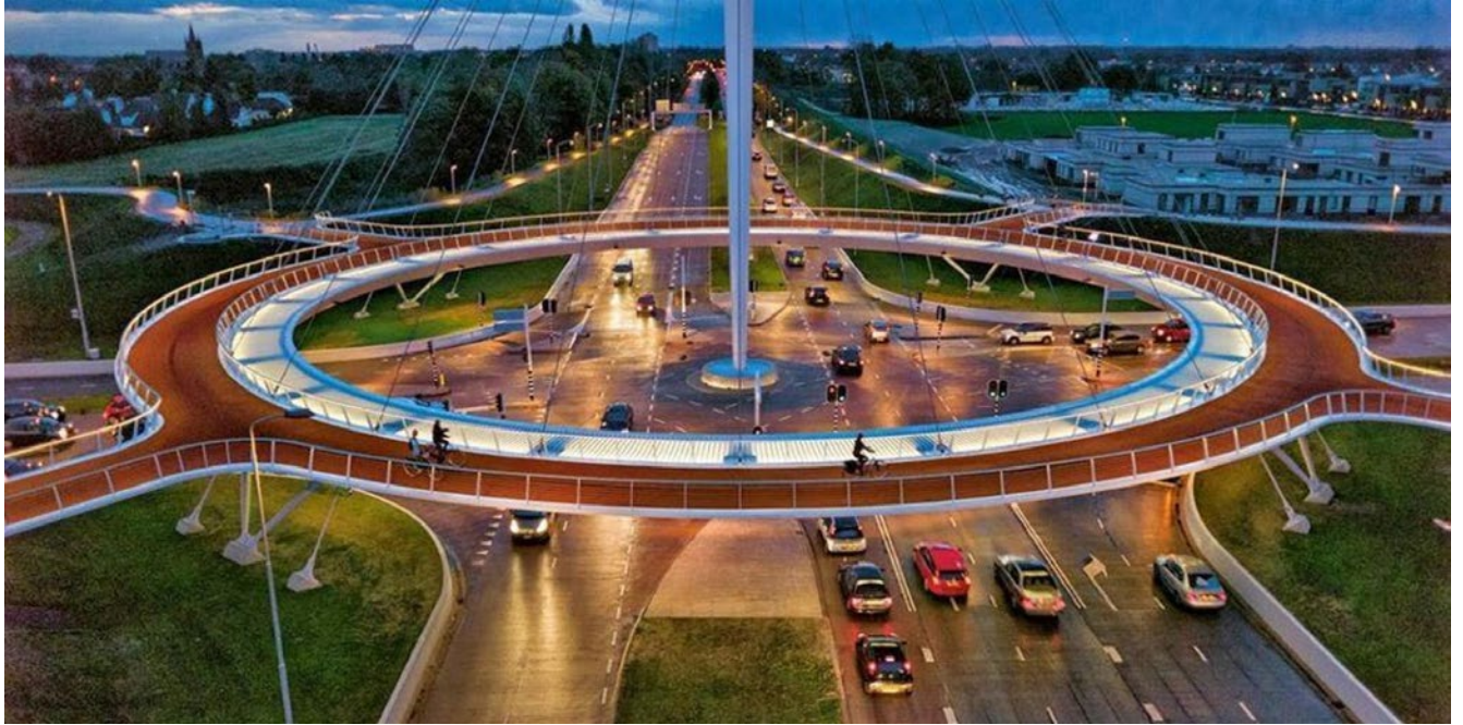
Figure 4-31 Hovenring Bridge traffic crossing
