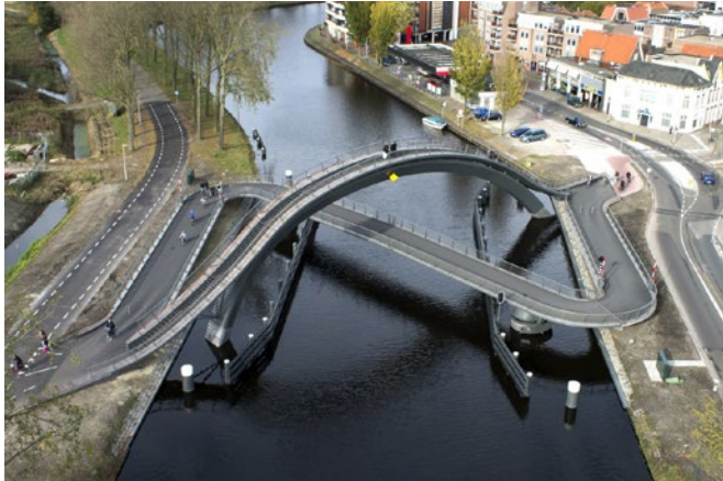
Figure 4-37 Melkwegbridge pedestrian and cyclist bridge aerial view
