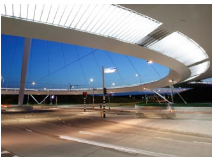
Figure 4-36 Hovenring Bridge intersection depression
