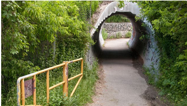
Figure 3-26 Rail Underpass near Bayview Ave. and DVP
