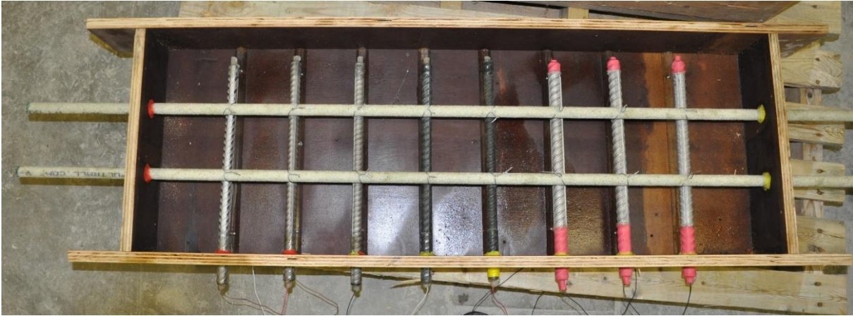
Figure 3-8: Formwork and bars for longitudinally cracked specimens
