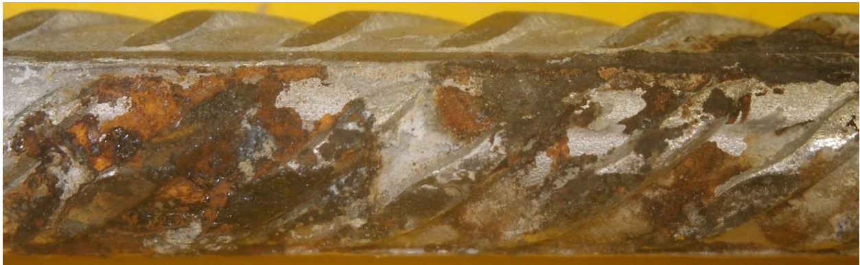
Figure 4-37: Delaminated corrosion product on 2101 stainless steel
