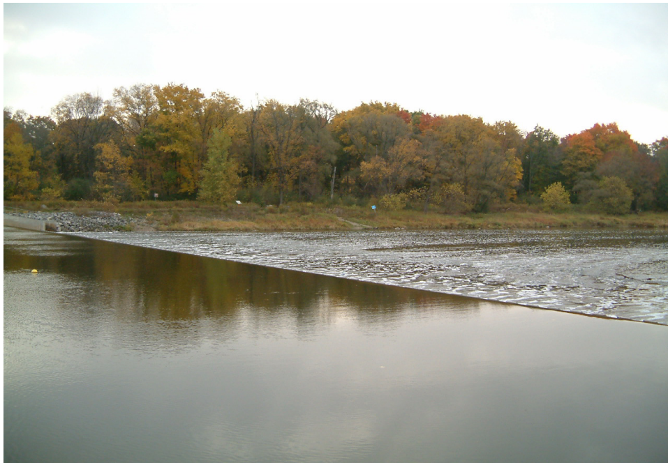
Figure 3.1: Raw Water Intake at Grand River
