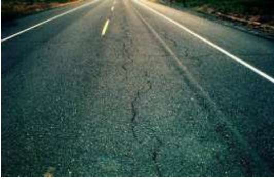
Figure 2-4: Longitudinal Cracking
