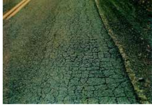
Figure 2-5: Fatigue Cracking
