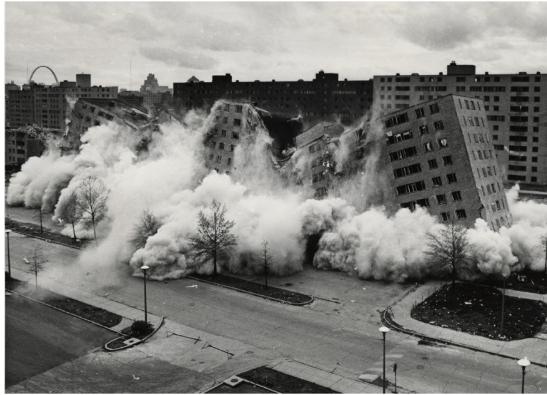
Fig. 1-37 The Demolition of Pruitt-Igoe
