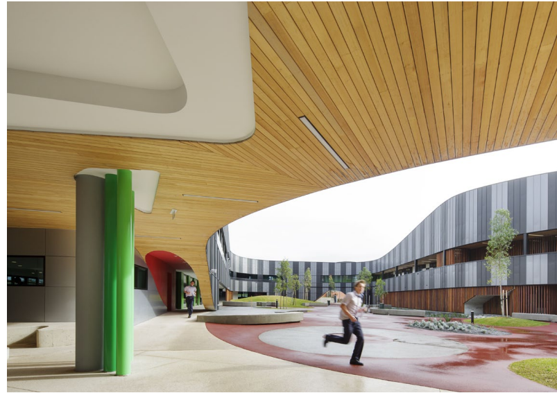
Fig 5.19: View to the courtyard
