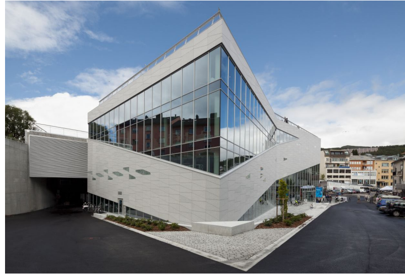
Fig 5.28: Exterior view of corner
