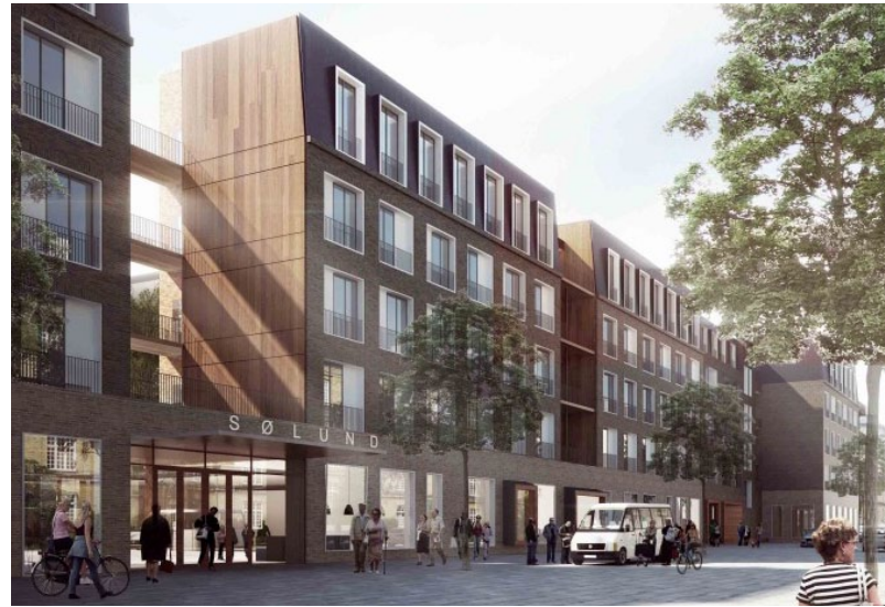
Fig 5.26: Exterior view retirement community
