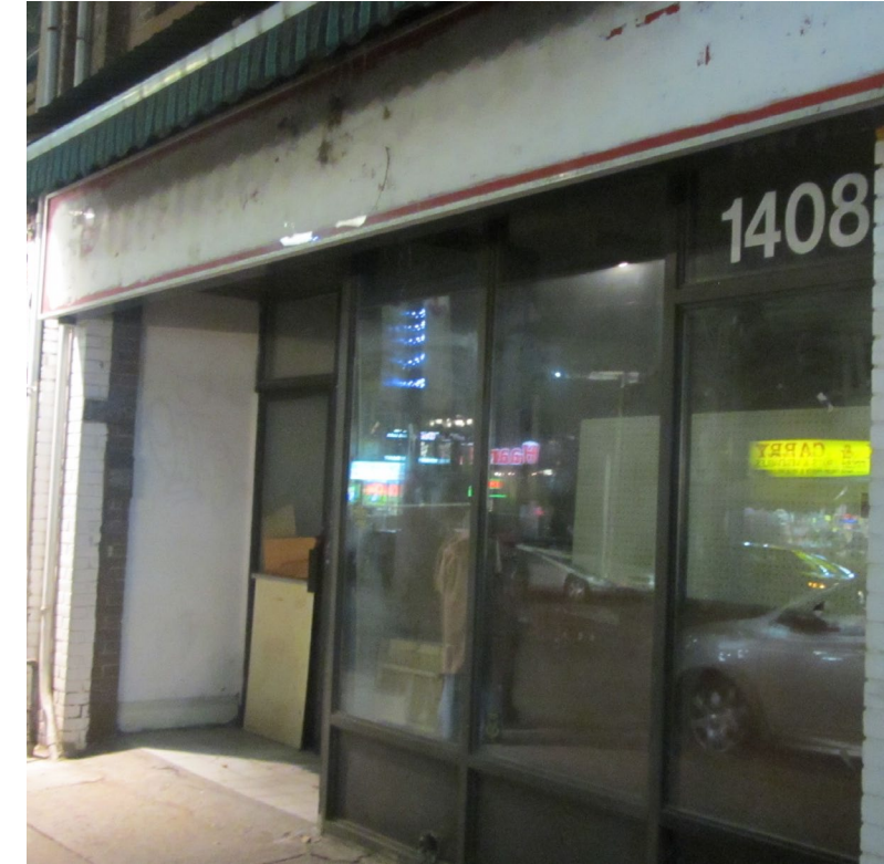
Fig 4.02: A vacant storefront within the Gerrard Bazaar
