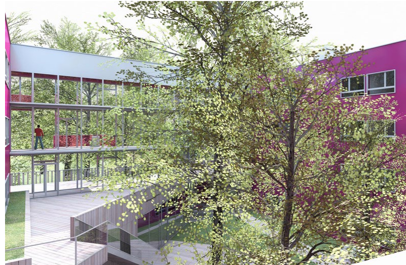
Fig 5.22: Courtyard view of senior residence
