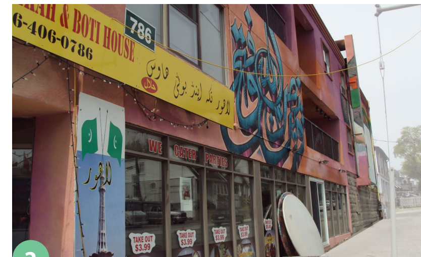
2 A mixed-use residential building is directly opposite the site which can compliment the senior residential complex
