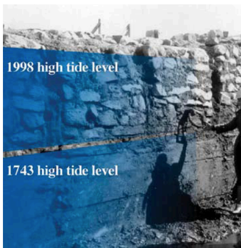
Figure 4.5: High tide marks at the Fortress of Louisbourg. (State of the Coast report 2009).
