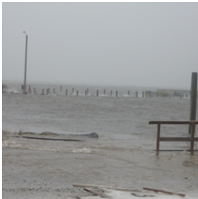
Figure 5.2: Flooding of Ingomar wharf in February 2013. (Photo courtesy of DFO-SCH).
