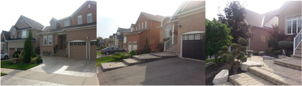
Figure 1.54: Example of entrances in Jefferson Forest Richmondhill
