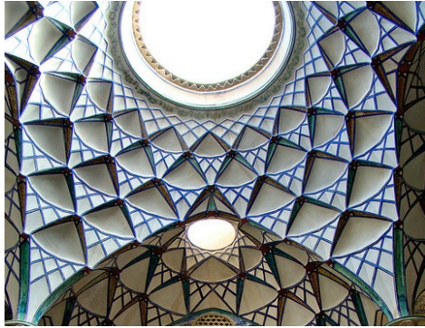
Figure 1.25: Brojerdi House-Details and openings in the main hall ceiling
