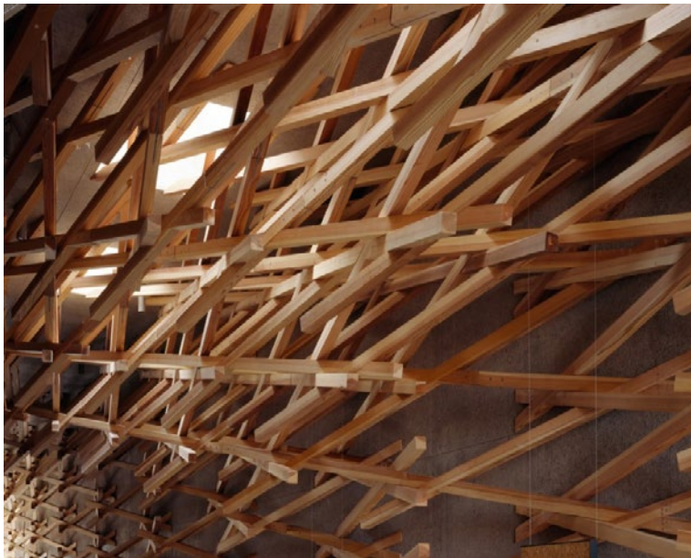
Figure 2.35: Starbucks café by Kengo Kuma & Associates, Dazaifu, Fukuoka Prefecture, Japan, Wood Structural System
