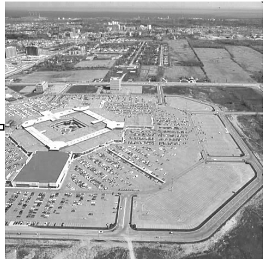
Figure 3.31:Square One Shopping Centre, Mississauga
