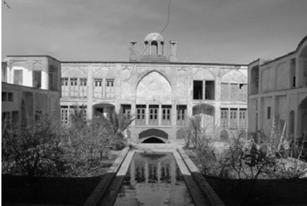
Sharifian House 1814 Figure 1.08: Sharifian House, court yard vignette,
