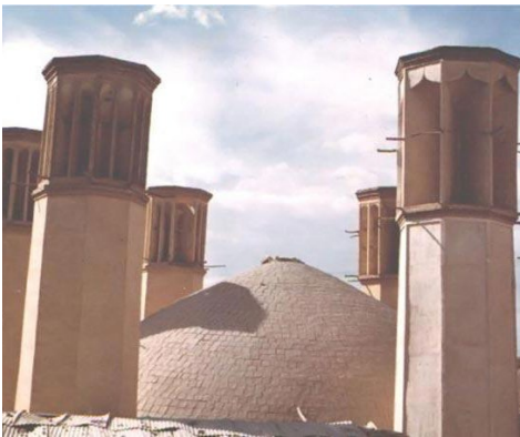
Figure 1.15: 6-Badgir-water reservoir in the world at the ancient Iranian city of Yazd
