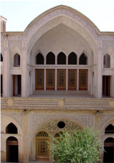
Figure 1.20: Brojerdi house southern balcony
