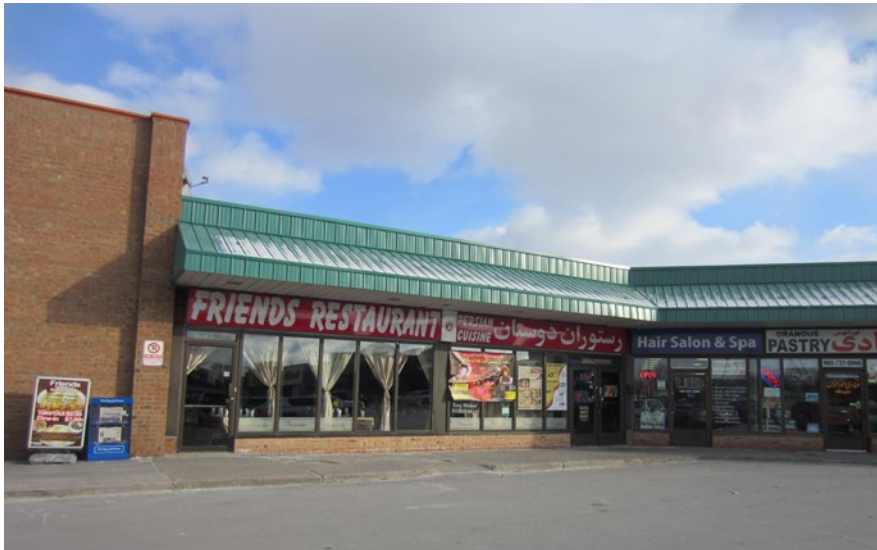
Figure 3.74: Existing Plazas, Yonge and 16th – Richmond Hill
