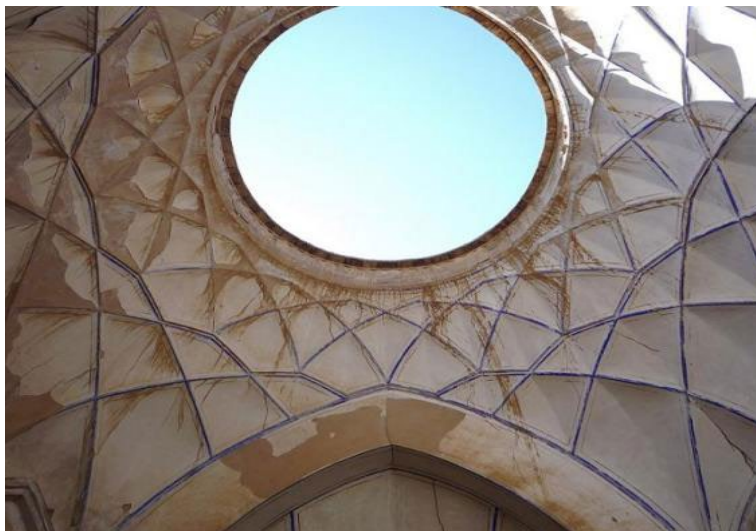
Figure 1.30:Sharifian House, char-safe- illustration of ceiling
