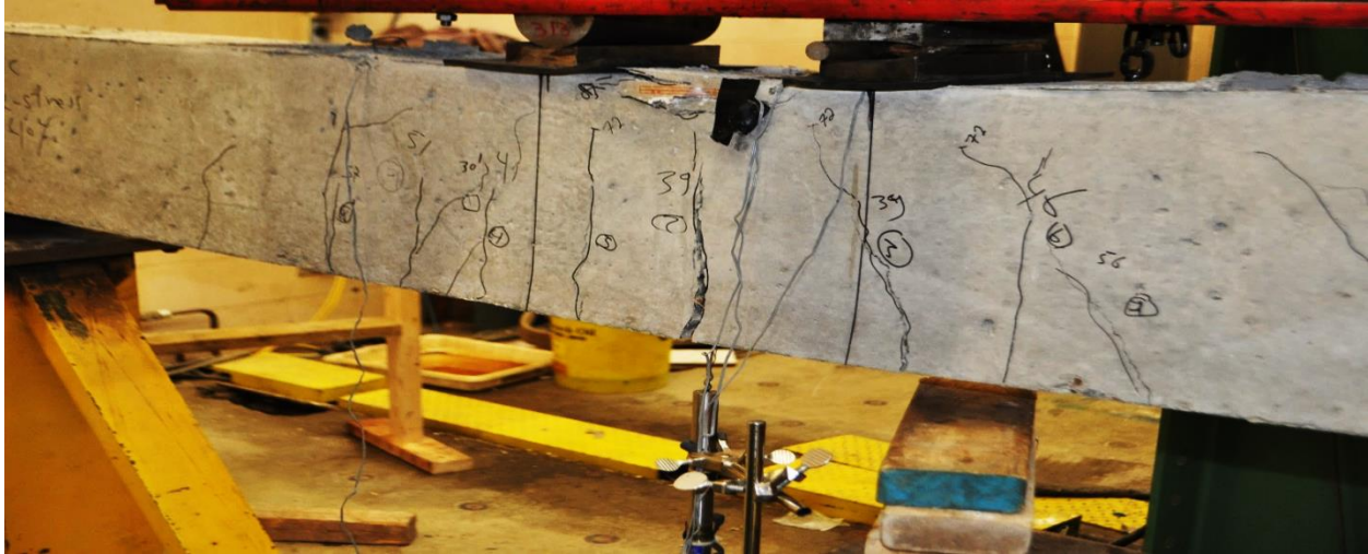
Figure 4- 6 Mode of failure of 40% prestressed beam under static loading
