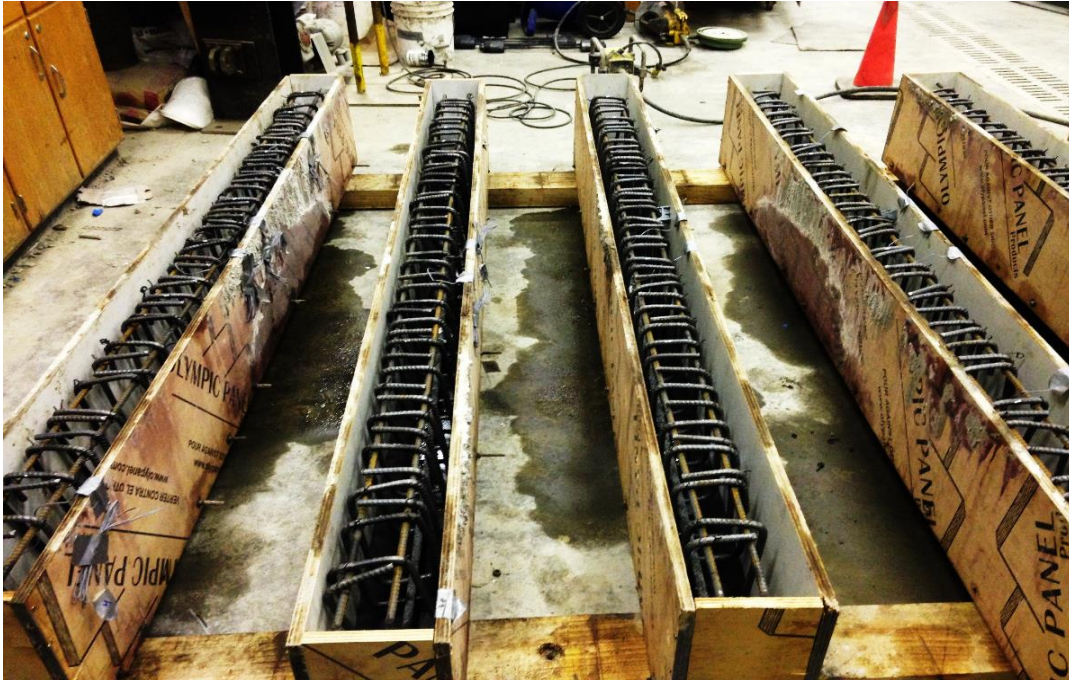
Figure 3- 5 Form work used to cast all the beam specimens
