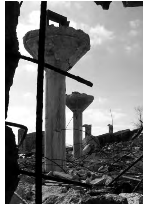
Figure 3.19: (above) Columns on the collapsing roof of building #92, the axle and transmission shops, 2012.
