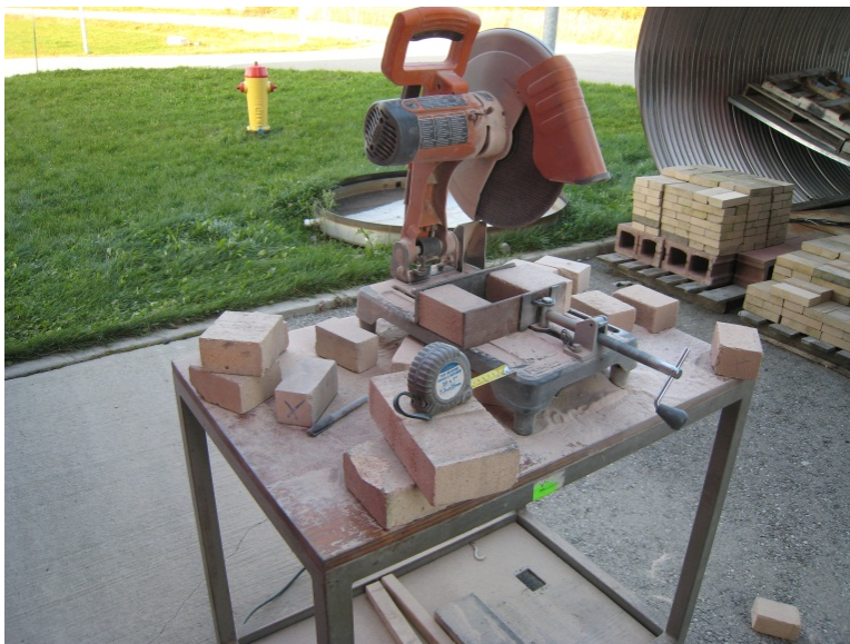
Figure A.5: Radial arm saw is used to cut fire bricks to size
