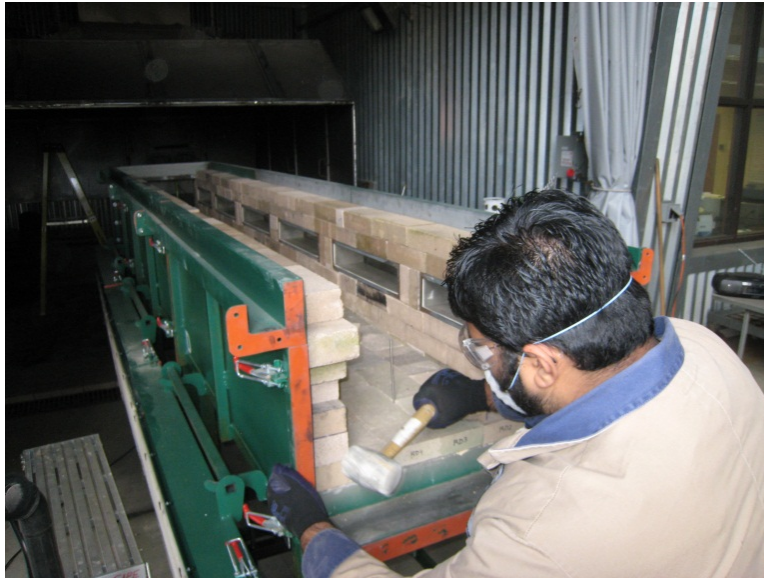
Figure A.8: Bricks are evenly aligned at the joints for a smooth transition between modules
