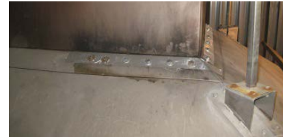
(b) Slanted flange-fume hood connection
