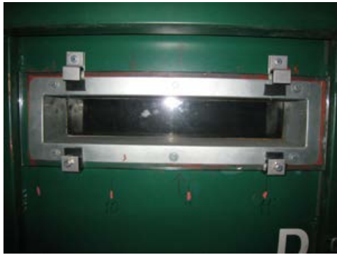
(a) Exterior window pane
