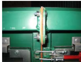
(b) Tight-seal joints
