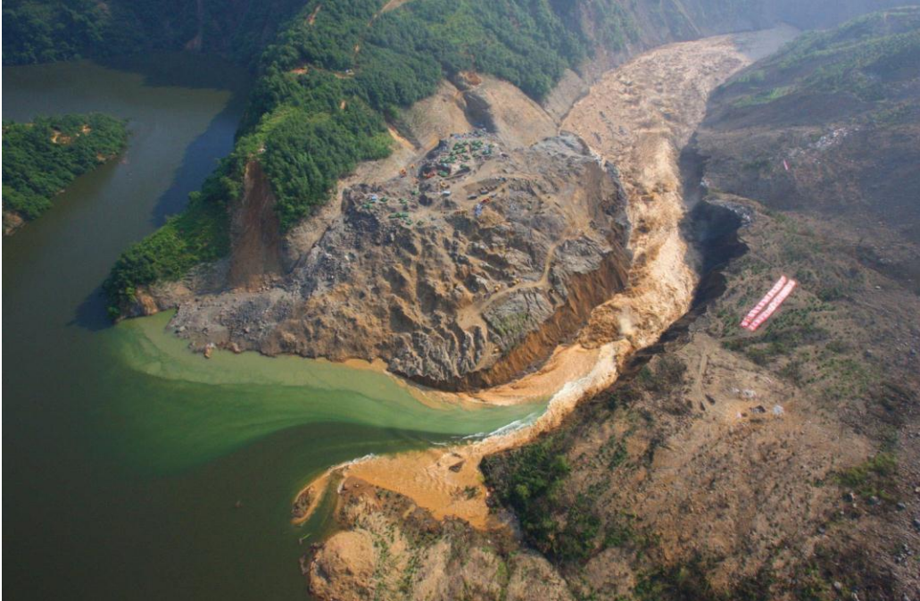
Figure 1.5. Tangjiashan landslide-dammed lake during controlled breach on June 10, 2008. Note the enlarged spillway caused by water incision over the landslide body (Photographed by Prof. Liu Ning. Figure 10.14 from Cui et al. 2011).
