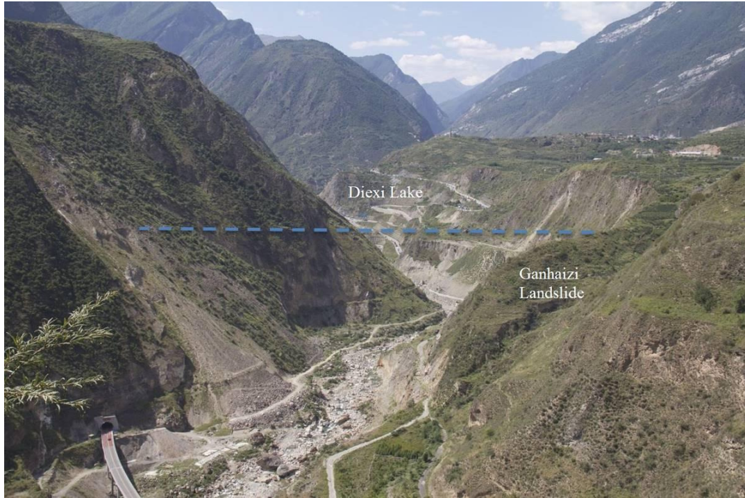
Figure 3.6. Photograph of the remnant dam of Diexi Lake, which was formed by the Ganhaizi landslide and the Diexi landslide (taken on 17/08/2013).
