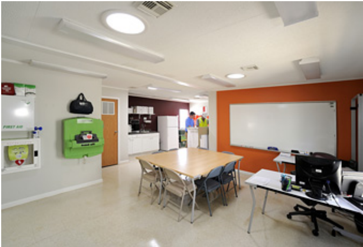
Figure 44 & 45: reMOD by Williams Scotsman and Skanska
