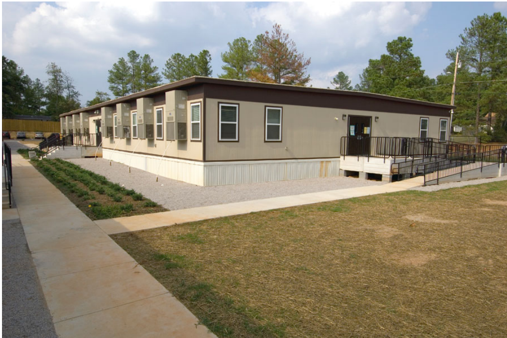
Figure 5: Portable Classrooms - ModSpace
