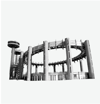
Fig 87. New York State Pavilion (1964) Philip Johnson
