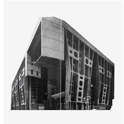
Fig 101. London Bank Buenos Aires (1966) Clorindo Testa
