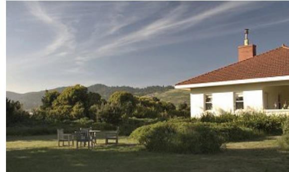
FIG. 3.13. Commonweal Retreat Center, Kohler House
