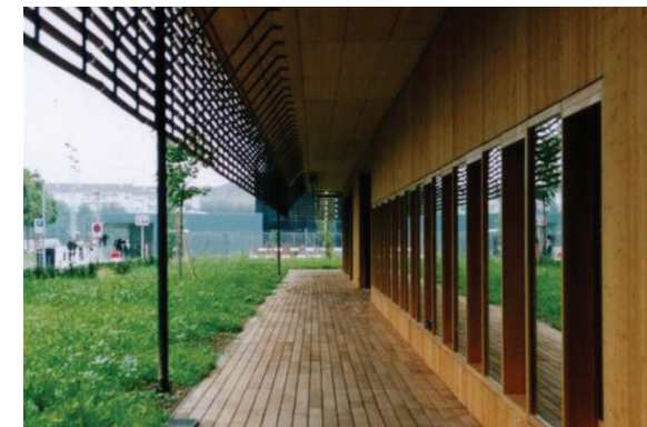
FIG. 4.11. Rehab Centre, Walkway
