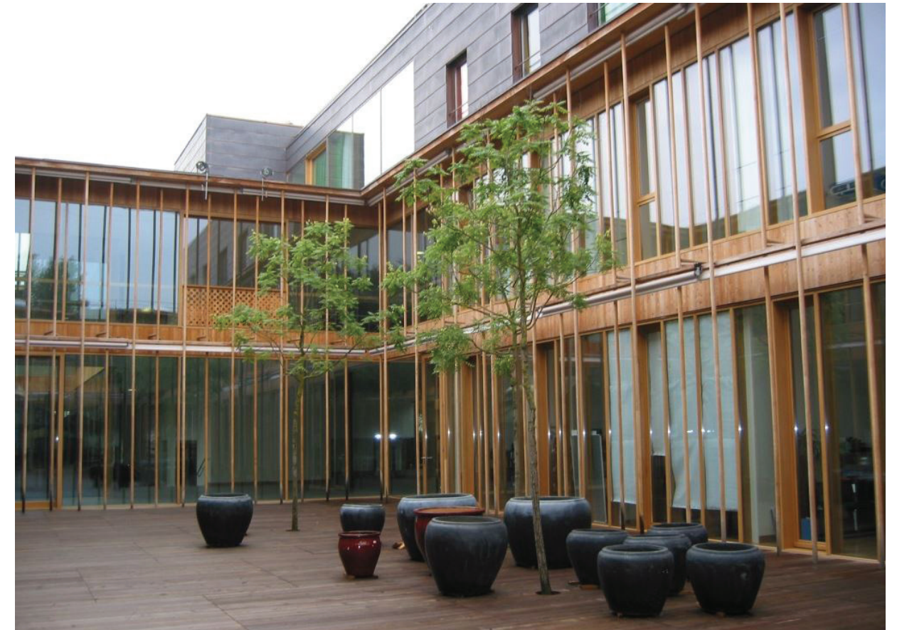
FIG. 4.10. Rehab Centre, Courtyard
