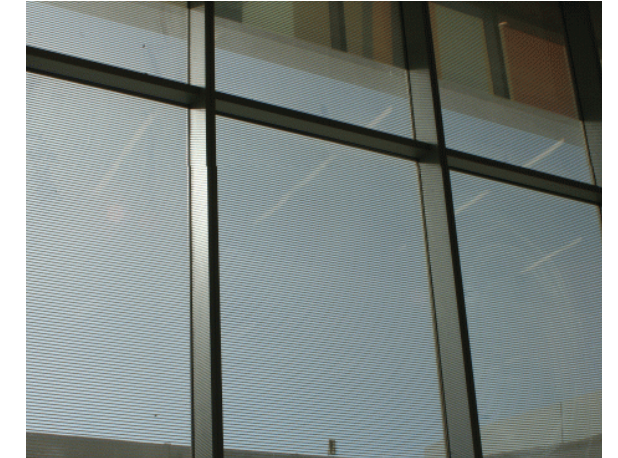
FIG. 4.17. “View Dynamic Glass” can stop light from penetrating through by the touch of a button, without the use of curtains.
