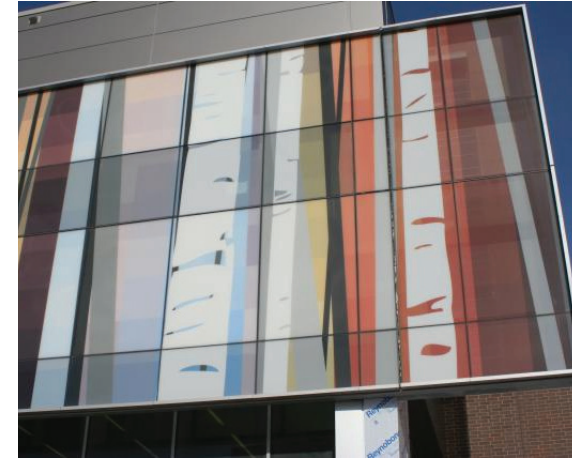
FIG. 4.16. Exterior view of the “View Dynamic Glass,” which carefully controls light penetration.
