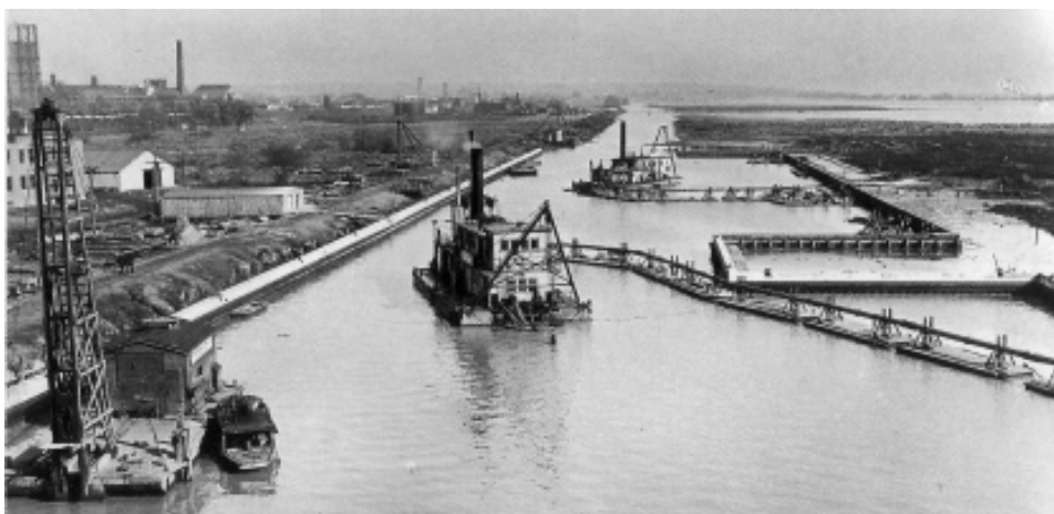
9c. "Hydraulic dredges deepen Keating Channel as dockwall construction progresses, October 31, 1914."
