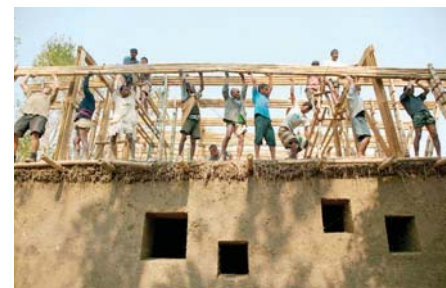
Fig. 2.14 Local laborers constructing METI Handmade School designed by Anna Heringer.
