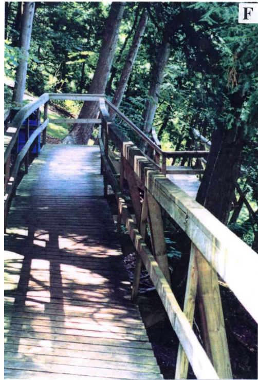
Surface F: Boardwalk
