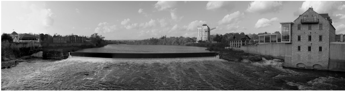
Figure 116: Parkhill Bridge Facing North
