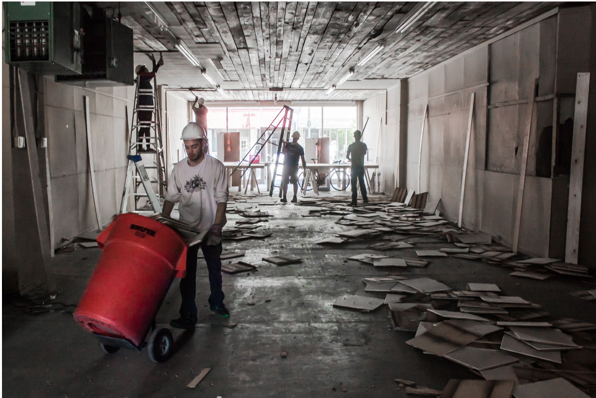
Plate 76: Removing ceiling tiles to expose barn board drop ceiling. [2015-06-06]
