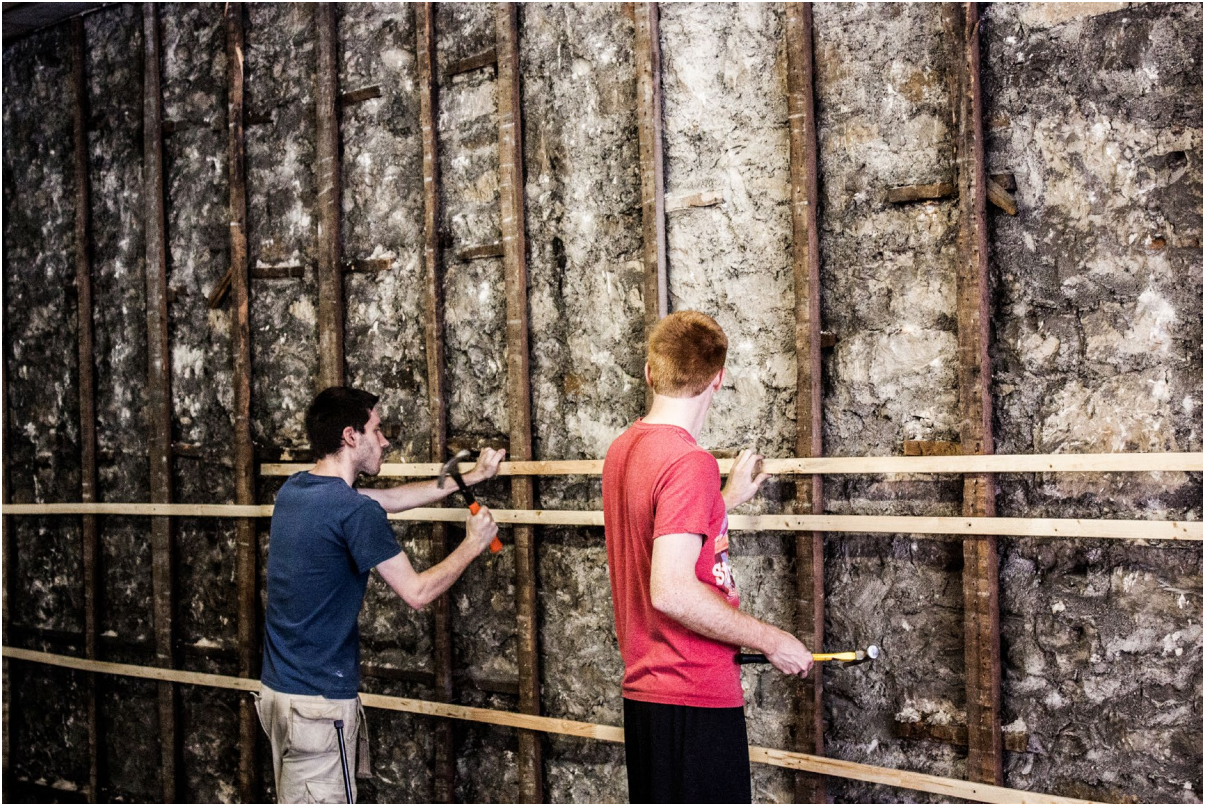
Plate 83: Installing strapping to mount drawings. [2015-07-15]
