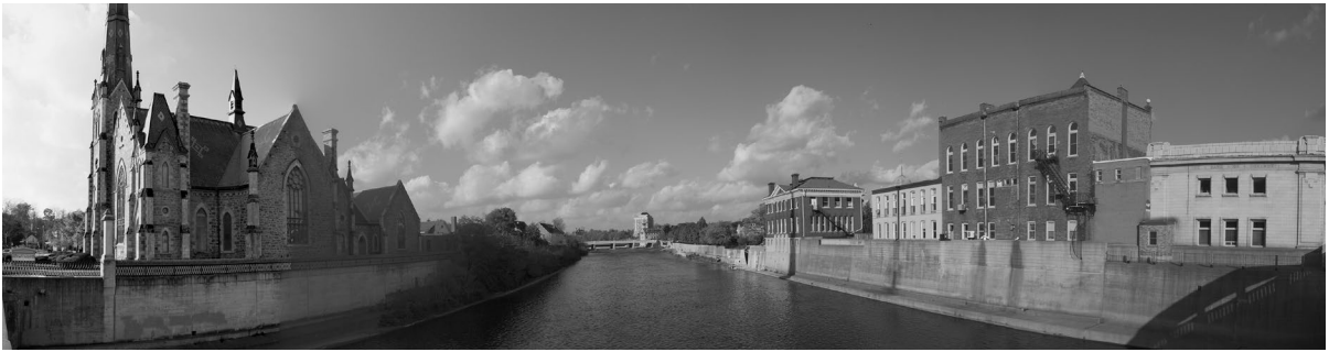
Figure 119: Main Street Bridge Facing North
