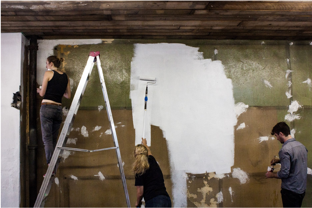
Plate 82: Painting the plaster wall. [2015-07-15]
