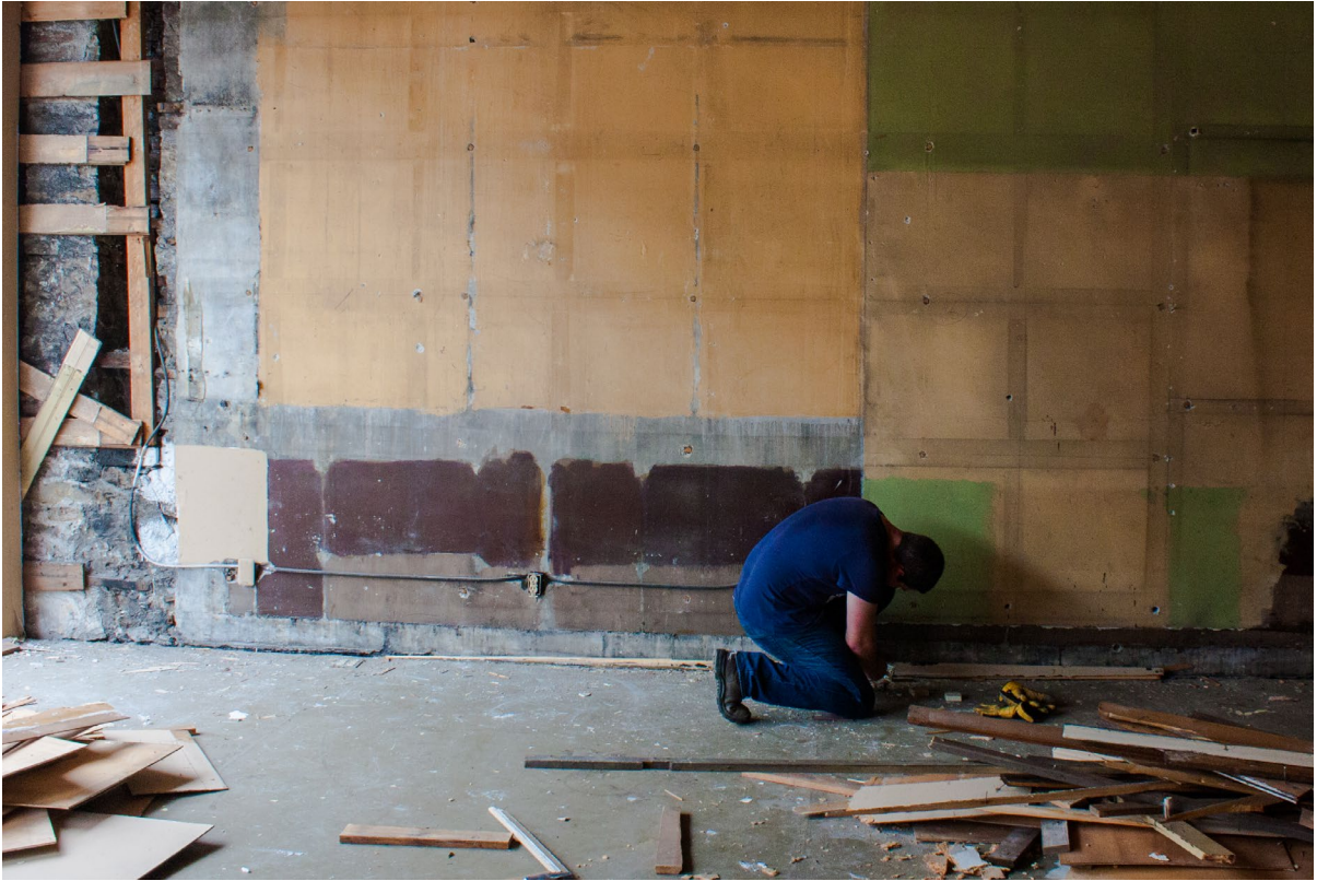
Plate 79: Carefully removing boards around the electrical conduit. [2015-06-27]
