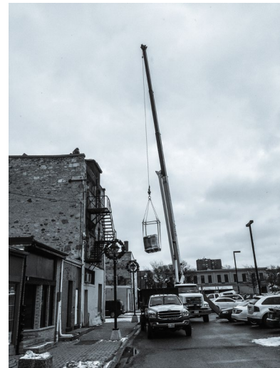
Figure 42: 35/37 Main Street roof repairs. [2014-11-28]
