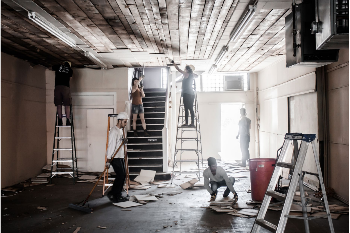
Plate 77: Removing ceiling tiles at the back of the storefront. [2015-06-06]
