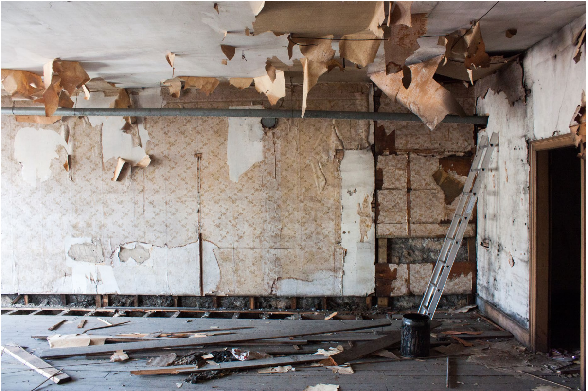
Plate 16: 39 Main Street second floor. [2015-06-26]
