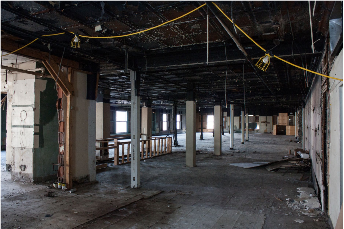
Plate 21: 60 Main Street Second Floor. [2015-06-26]
