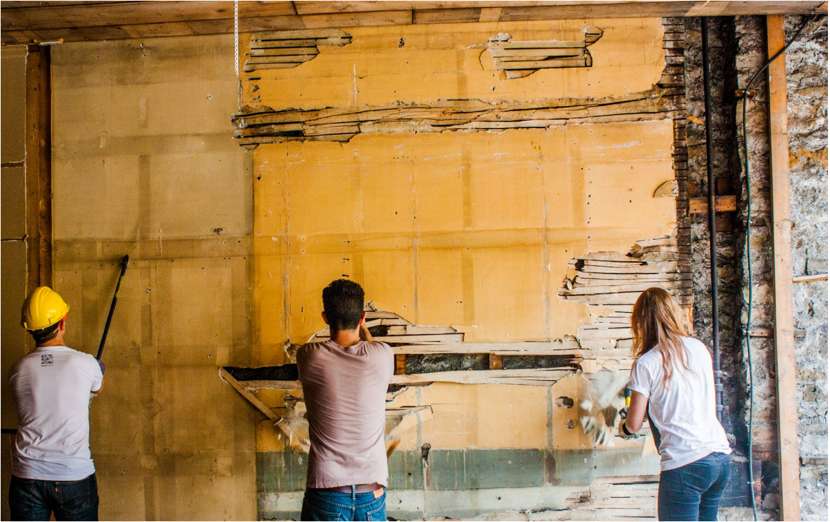
Plate 81: Demolishing the lath and plaster wall covering. [2015-07-05]
